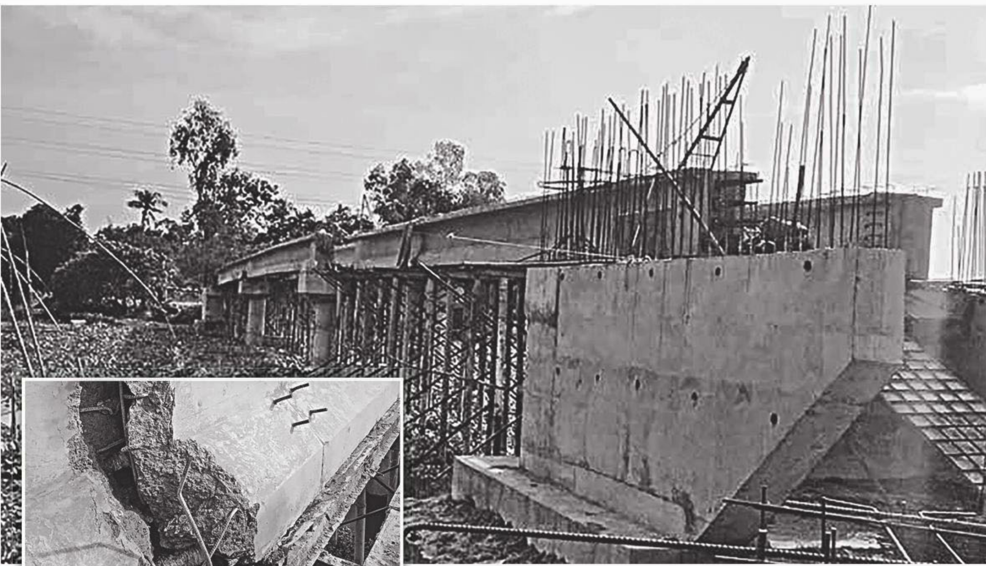
A girder of an under-construction bridge in Tangail's Ghatail upazila lies broken.
