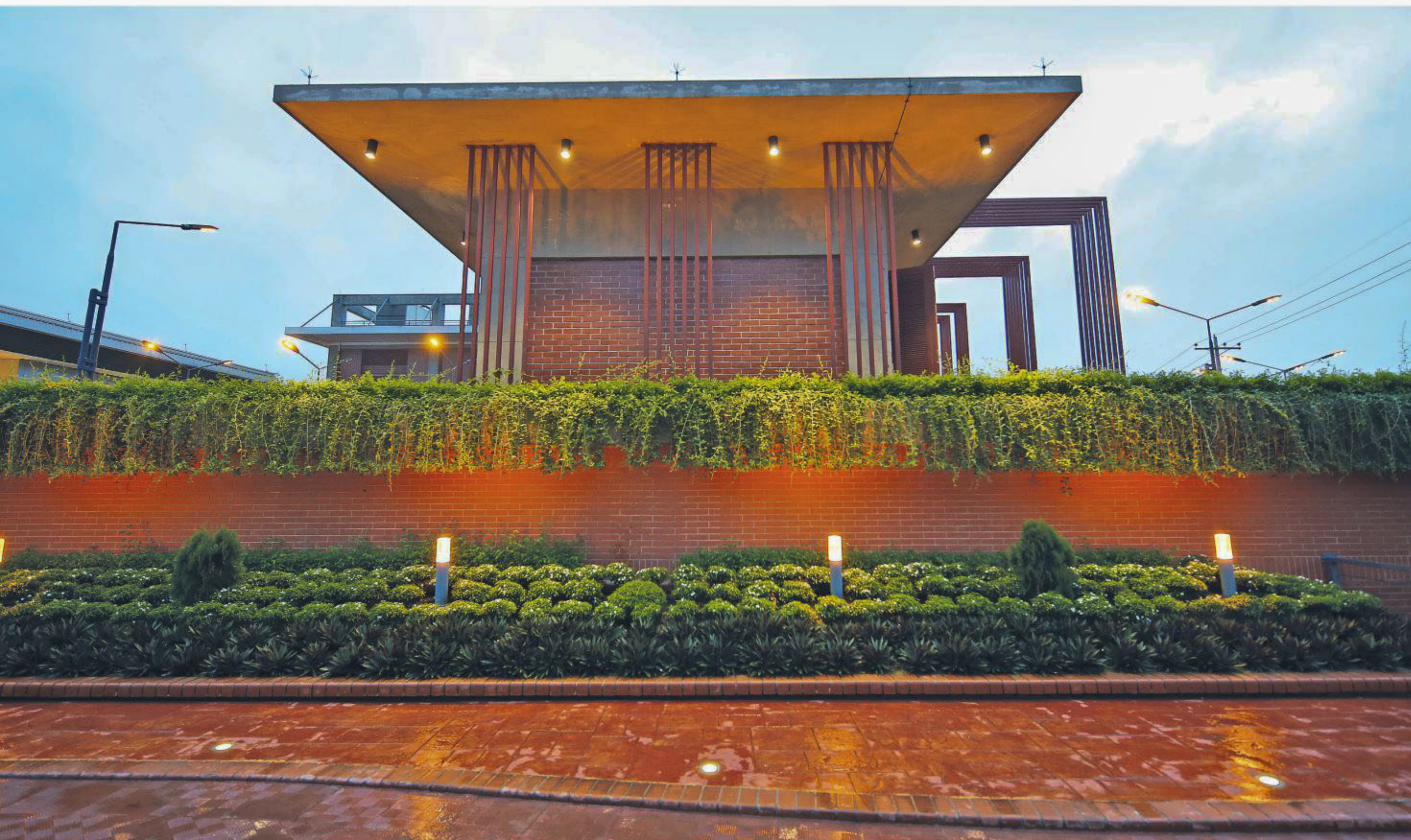
The Columbia Washing Plant in Gazipur.
