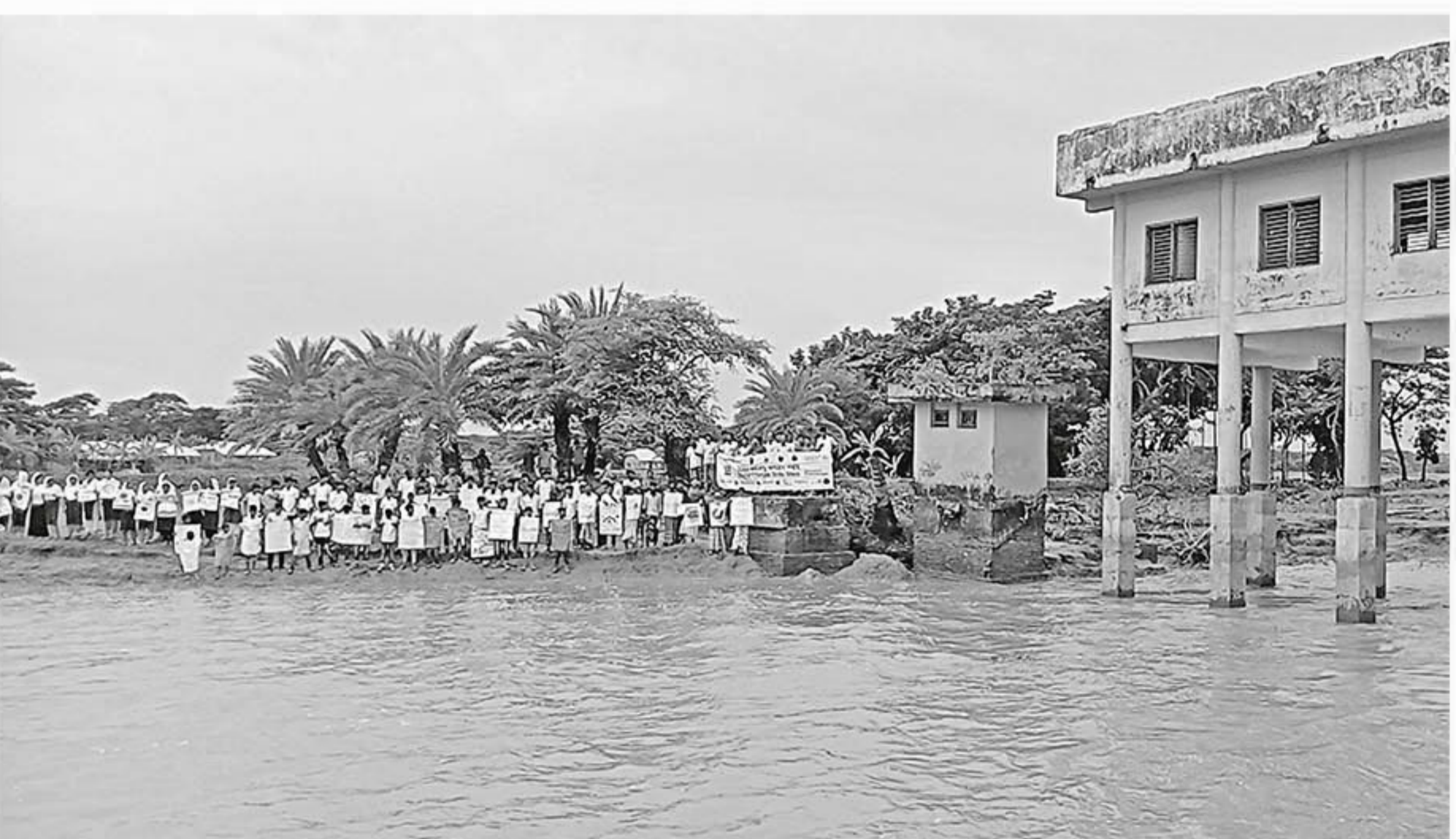
People form a human chain in front of a vulnerable cyclone shelter on the Ramnabad river in Chalitabunia union under Rangabali upazila on Wednesday demanding steps for protection against erosion to save their dwellings, agricultural lands and different set-ups in the area.
