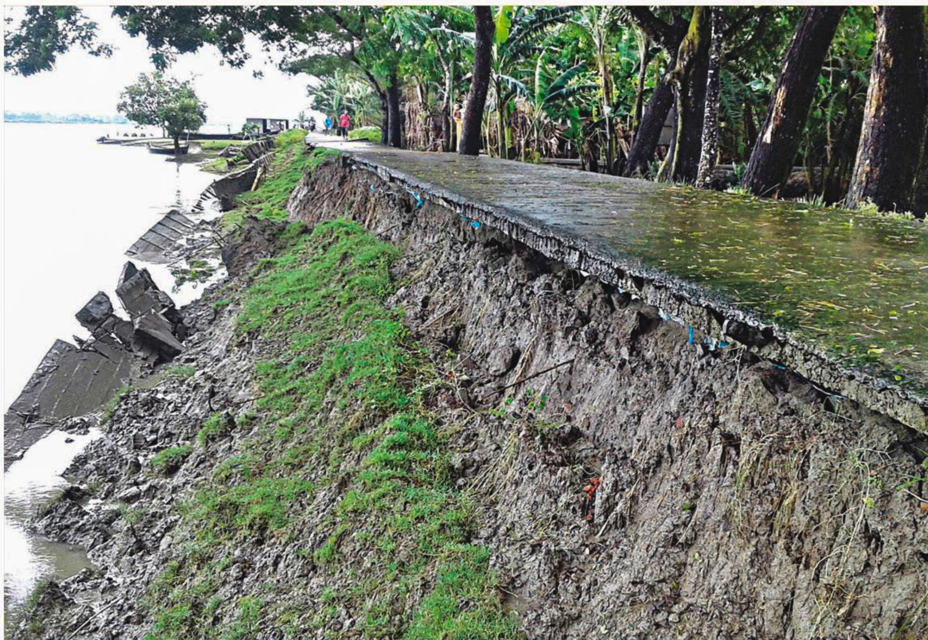
Part of the Kalapara-Kuakata Bikalpa Sarak is being eroded by the Sonatola river in Patuakhali's Tegachhia Bazar area. About 50 metres of the boundary wall, put up to protect the road, collapsed recently. The Local Government Engineering Department had built the wall and repaired the road only a year ago. The photo was taken on Thursday.
