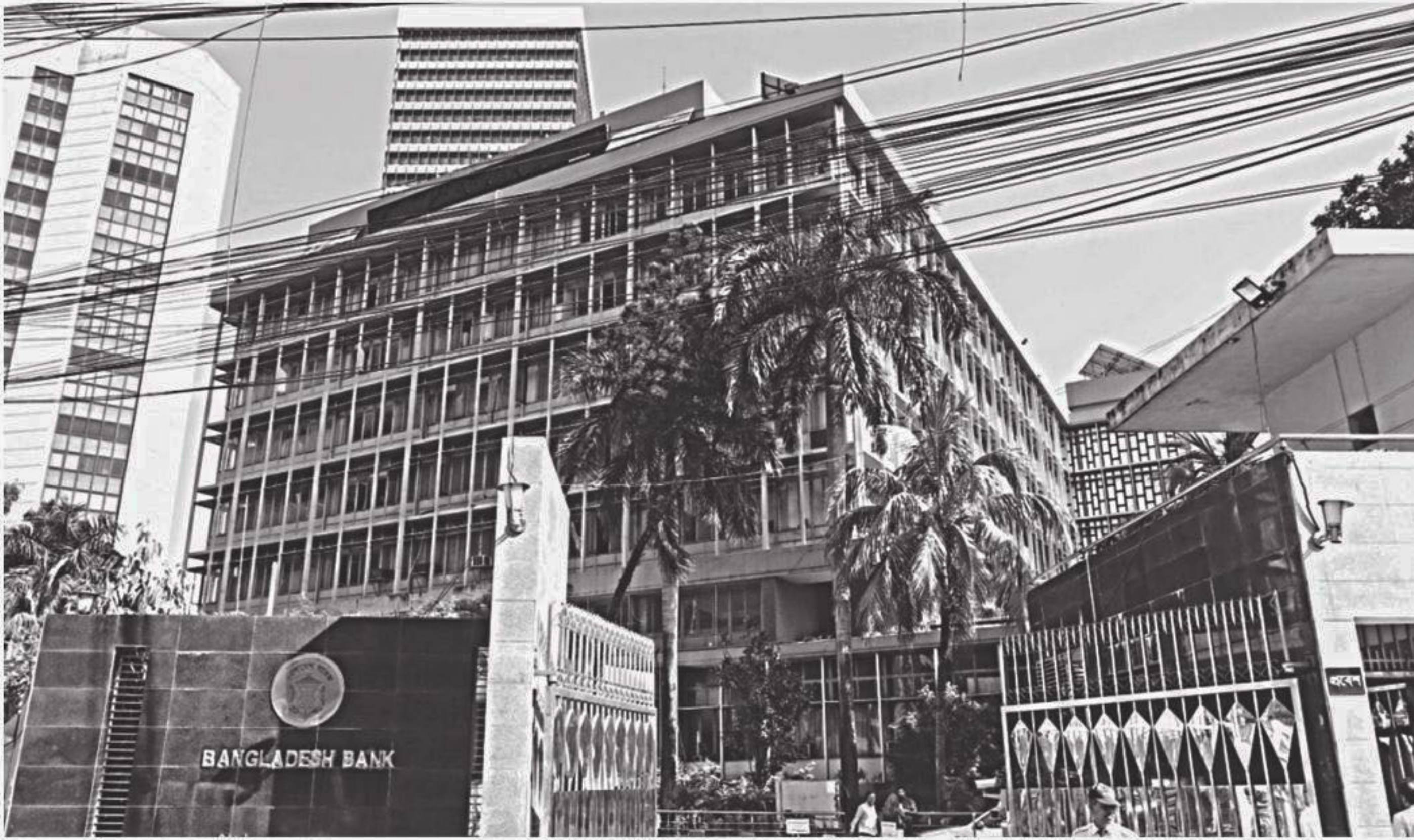
The Bangladesh Bank headquarters in Dhaka.
