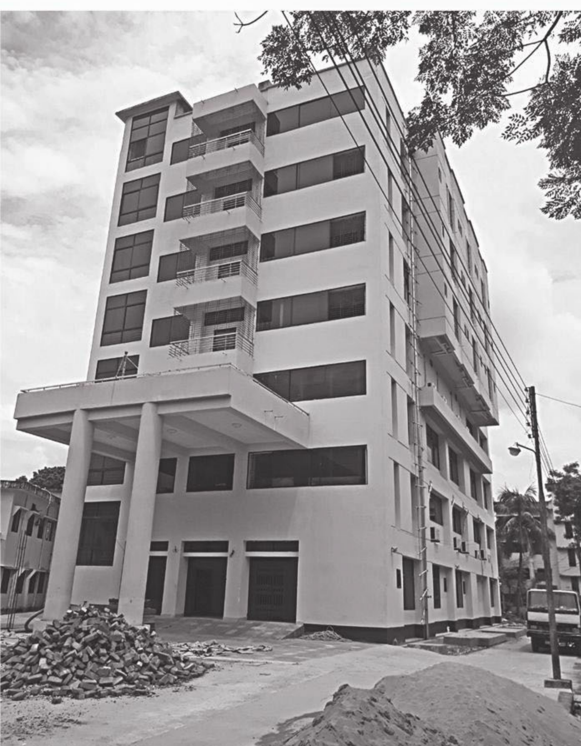
Newly built 250-bed Thakurgaon Sadar Hospital.
