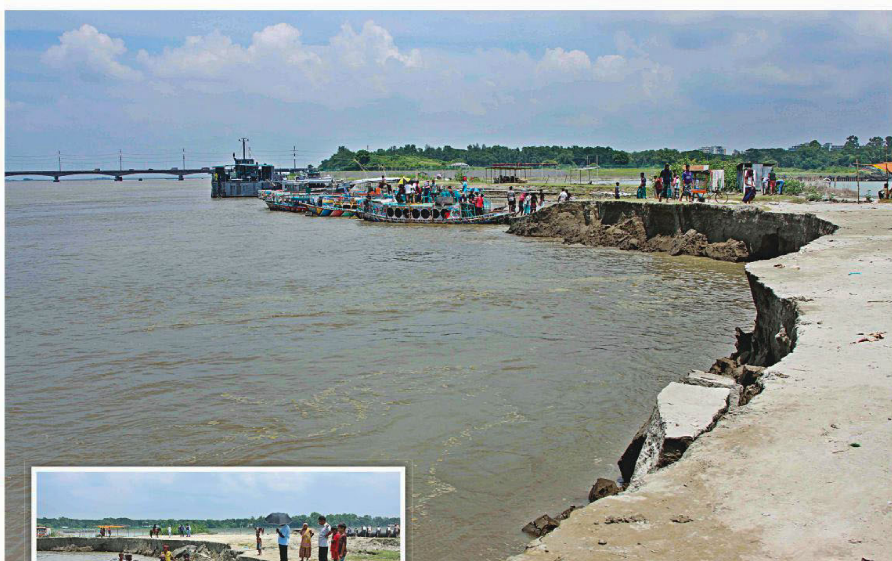
The Jamuna devours land at the harbour point near the Bangabandhu Multipurpose Bridge in Tangail yesterday. Locals see indiscriminate sand extraction from the river bed with powerful dredgers as one of the main reasons for the erosion. Inset, sand bags being dumped in the area to check the erosion.
