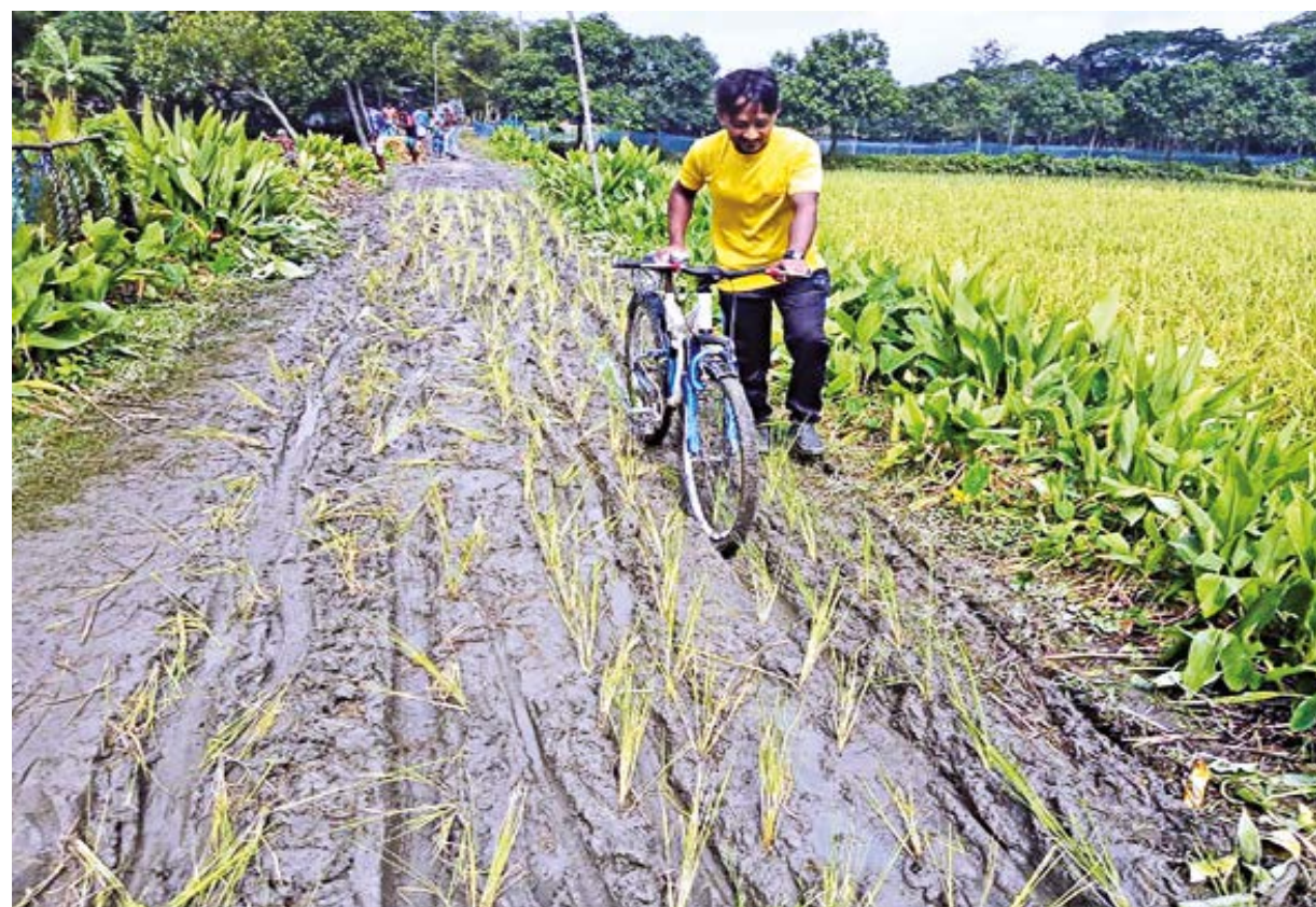
A NOVEL PROTEST: Villagers have planted paddy saplings on this mud road in Razibpur union of Ishwarganj upazila of Mymensingh, apparently in a bid to draw the attention of the authorities concerned as the three-kilometre way from Kashiganj to Momrempur remains a nuisance for people of five villages in the area.
