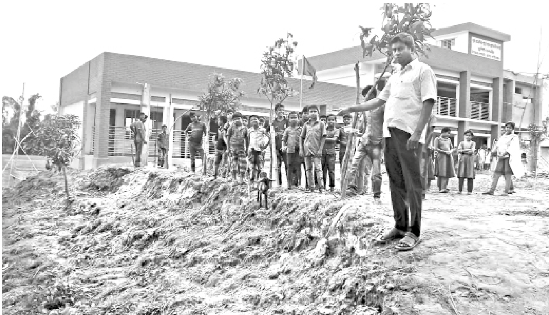
Amadirpara Government Primary School is one of the 43 institutions badly affected by the recent flood in Saghata upazila of Gaibandha.
