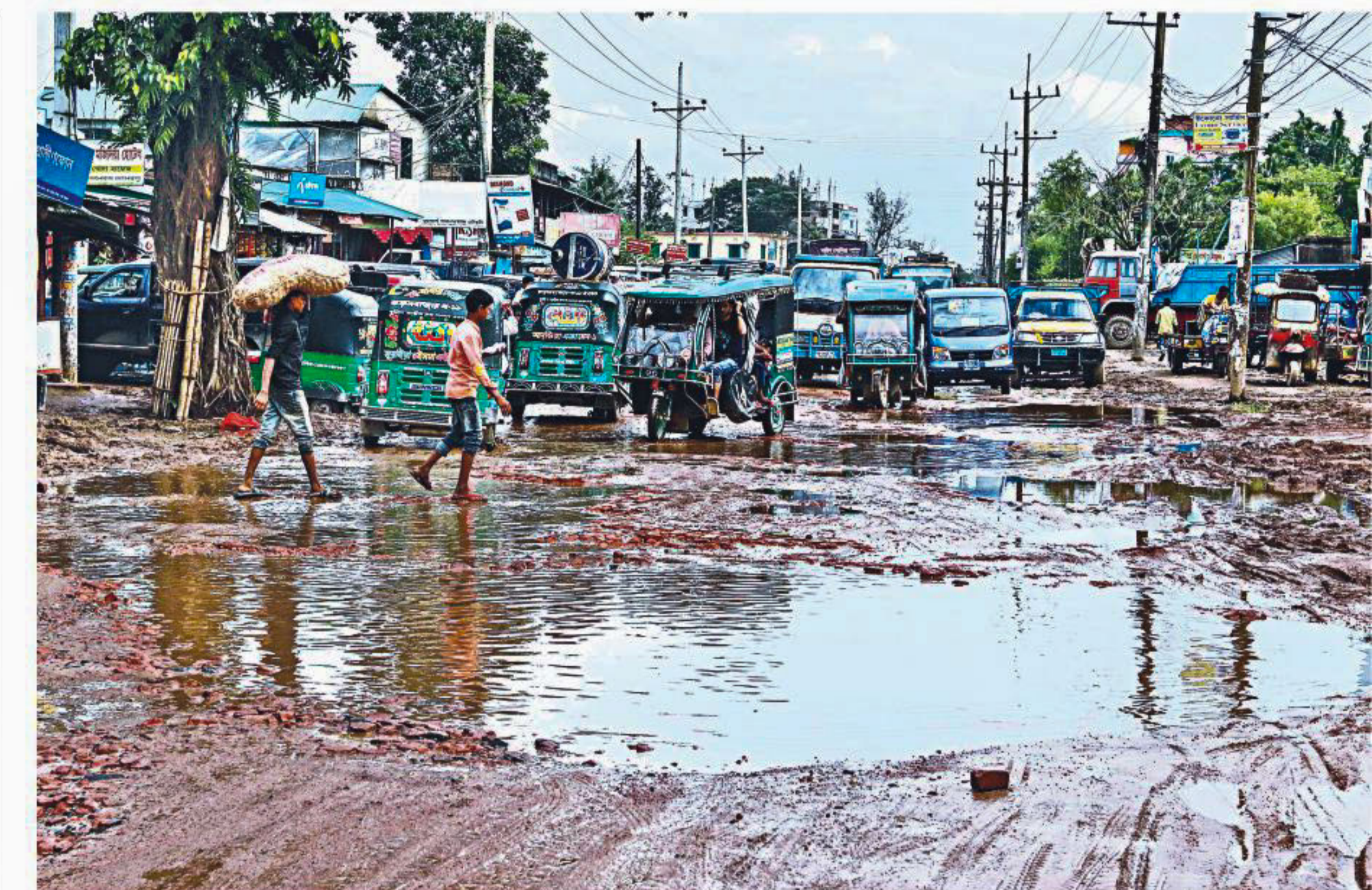
With potholes the size of small swimming pools scattered all over the road, commuting from Cox's Bazar to Teknaf has become a nightmare. This road is not just used by locals or tourists, vehicles of different government and aid agencies also have to ply it to reach Kutupalong refugee camp. The photo was taken from Court Bazar area of Cox's Bazar recently.
