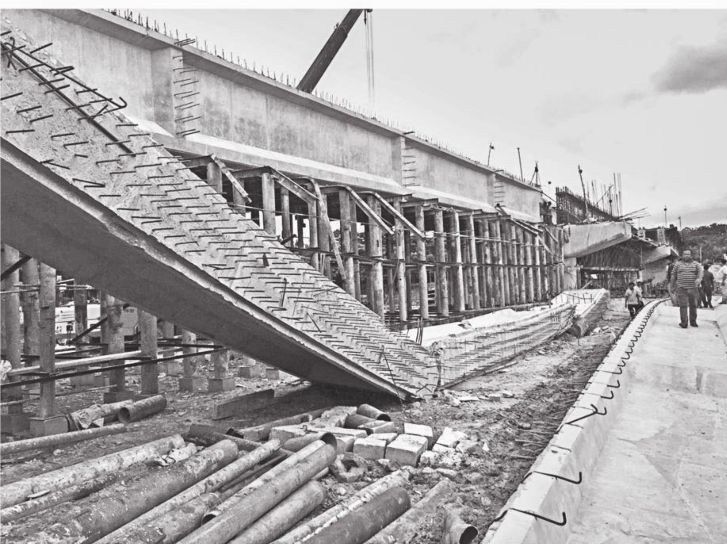
A couple of 100-foot-long girders of an under-construction bridge in Dhophagata area of Jhenidah Municipality tumbled down on Sunday. The Tk 120-crore bridge is being constructed by Japan International Cooperation Agency (Jica). Fortunately, there has been no casualties as all 20 workers at the site were at lunch when the incident took place.
