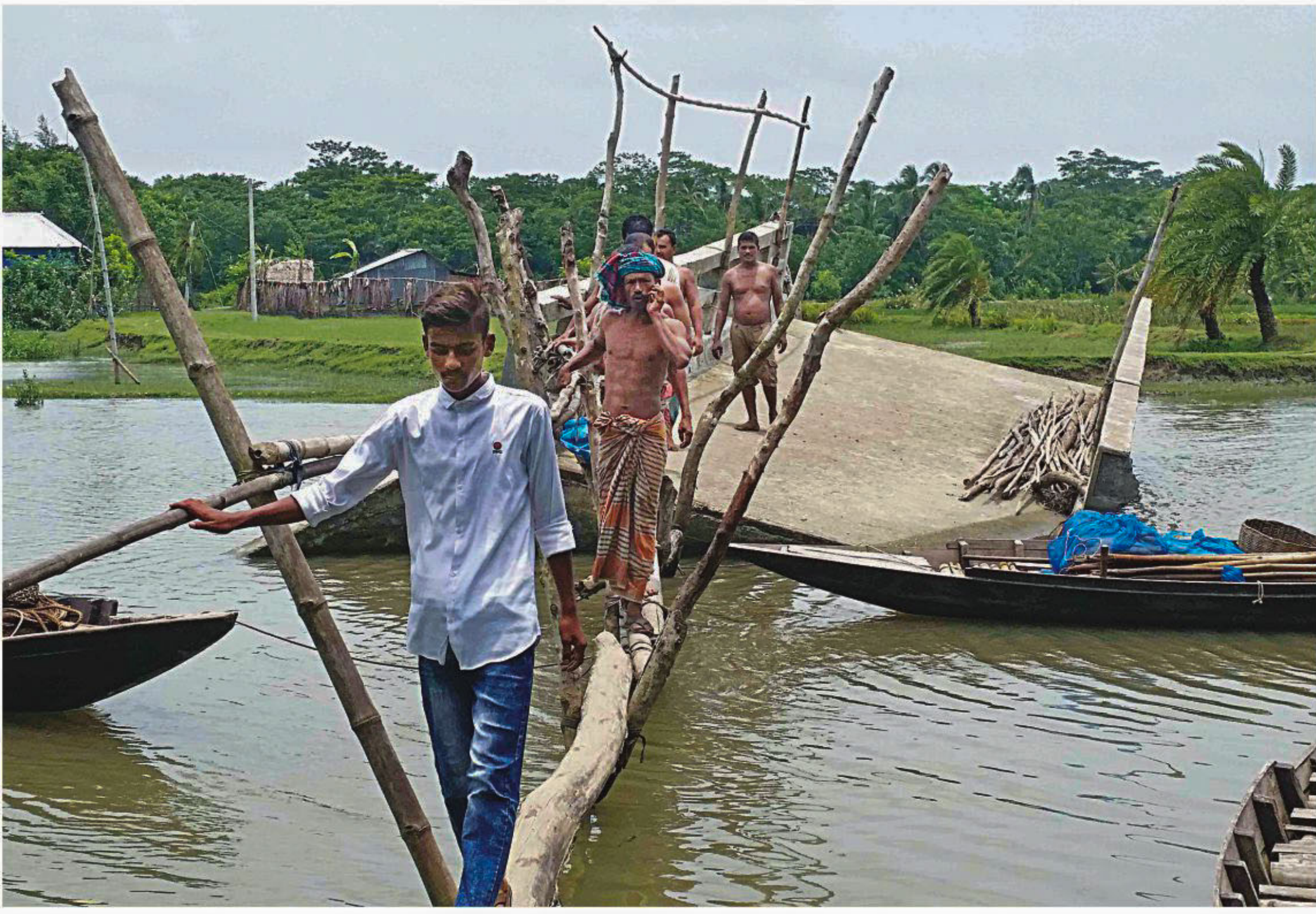
People cross a makeshift draw bridge over the Dafar-ara canal in Alokdia Vatchala area of Bagerhat. The approach road for the leaning concrete bridge was washed away in 2008, months after it was constructed. The bridge also started leaning around the same time.
