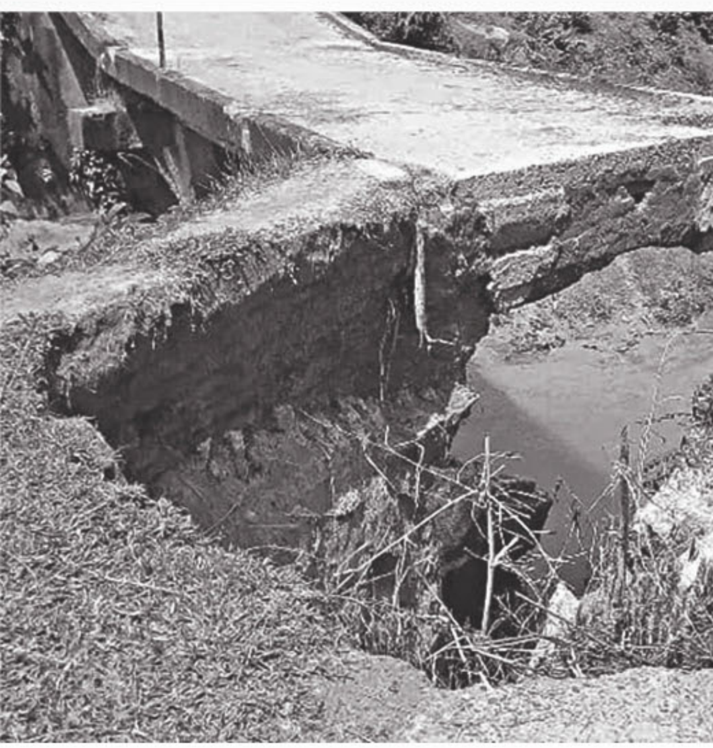
After the guide wall of the bridge on Baramchal-Munshibazar road in Kulaura gave way three days ago, its approach road also subsided, creating a gaping hole. PHOTO: MINTU DESHWARA
