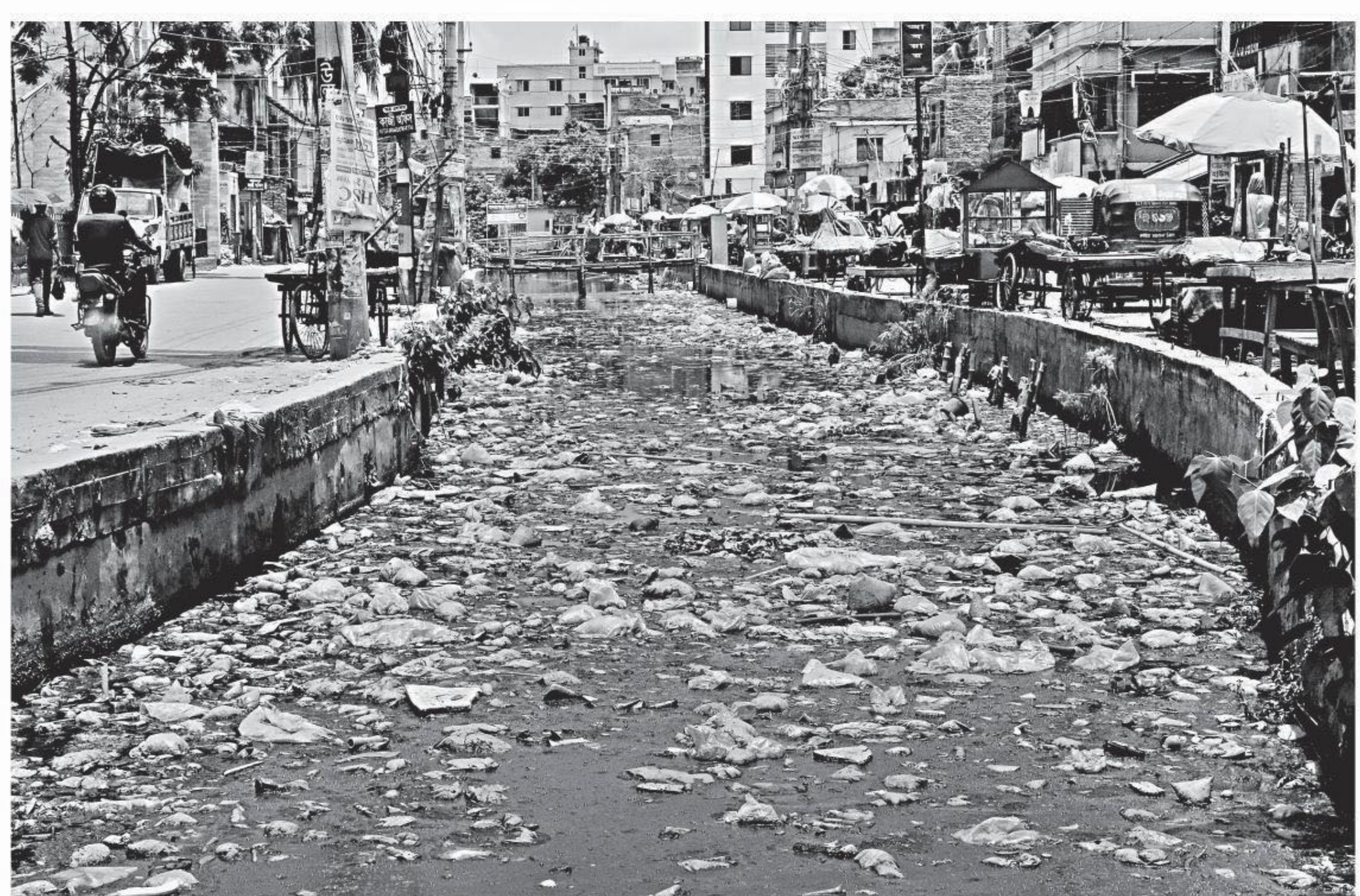
A SENSELESS ACT... Deb Dholaiakhal in Jurain has gone through a lot over the years. The canal has been shrunk to a narrow drain. It is also clogged up in many parts due to indiscriminate dumping of waste. The authorities concerned in an effort to save the waterbody cleaned it last month, but people have started using it as a dumping zone again. The photo was taken recently.
