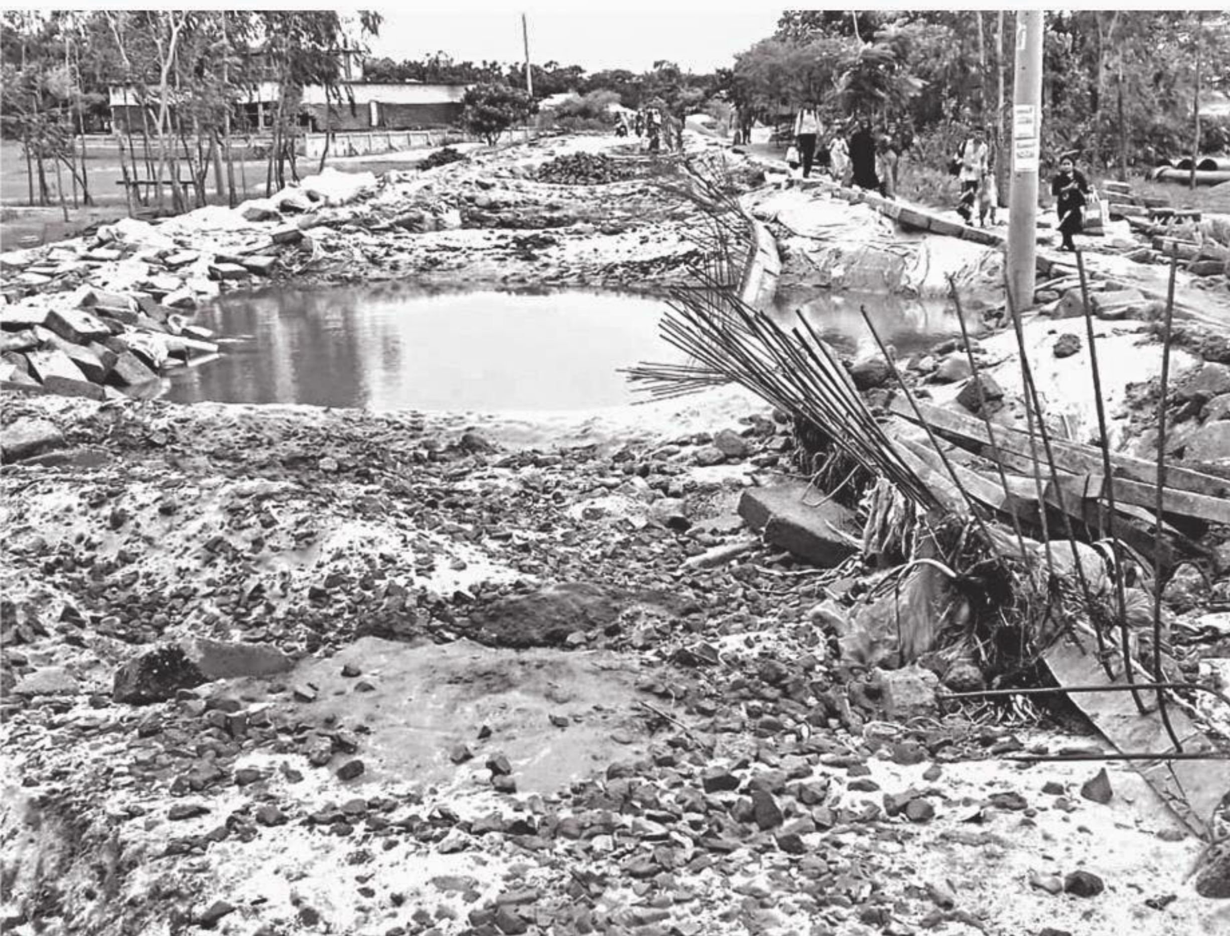
With upper asphalt layer completely washed away and large craters and potholes developed all over, this is what's left of the Sunamganj-Tahirpur road after the flood. The photo was taken in Tahirpur upazila recently.
