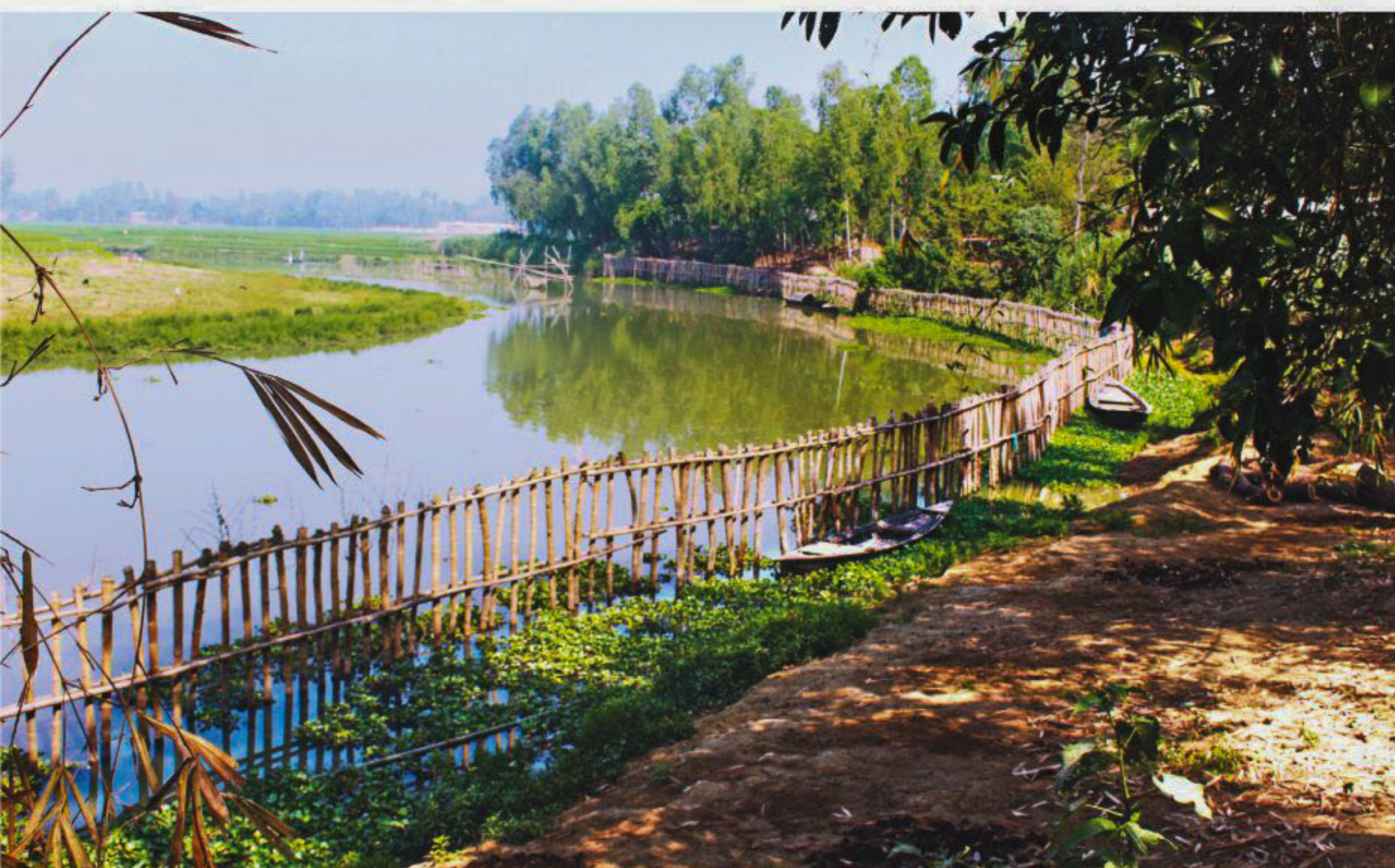
These bundals in Rowmari upazila were constructed defectively parallel to the bank instead of 45 degree curve, resulting in weakness of the structure and blocking access to the river.
