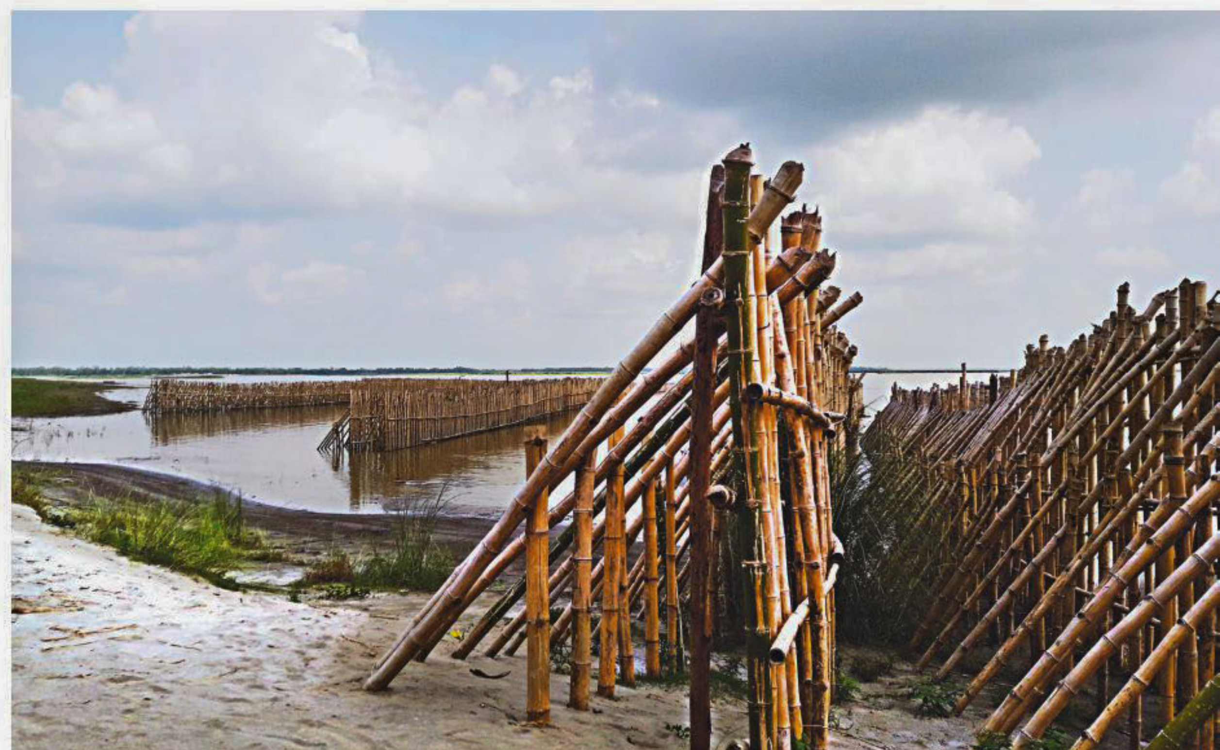
Bundals reduce river erosion by increasing sediment deopsit on the banks and by dredging the riverbed naturally.
