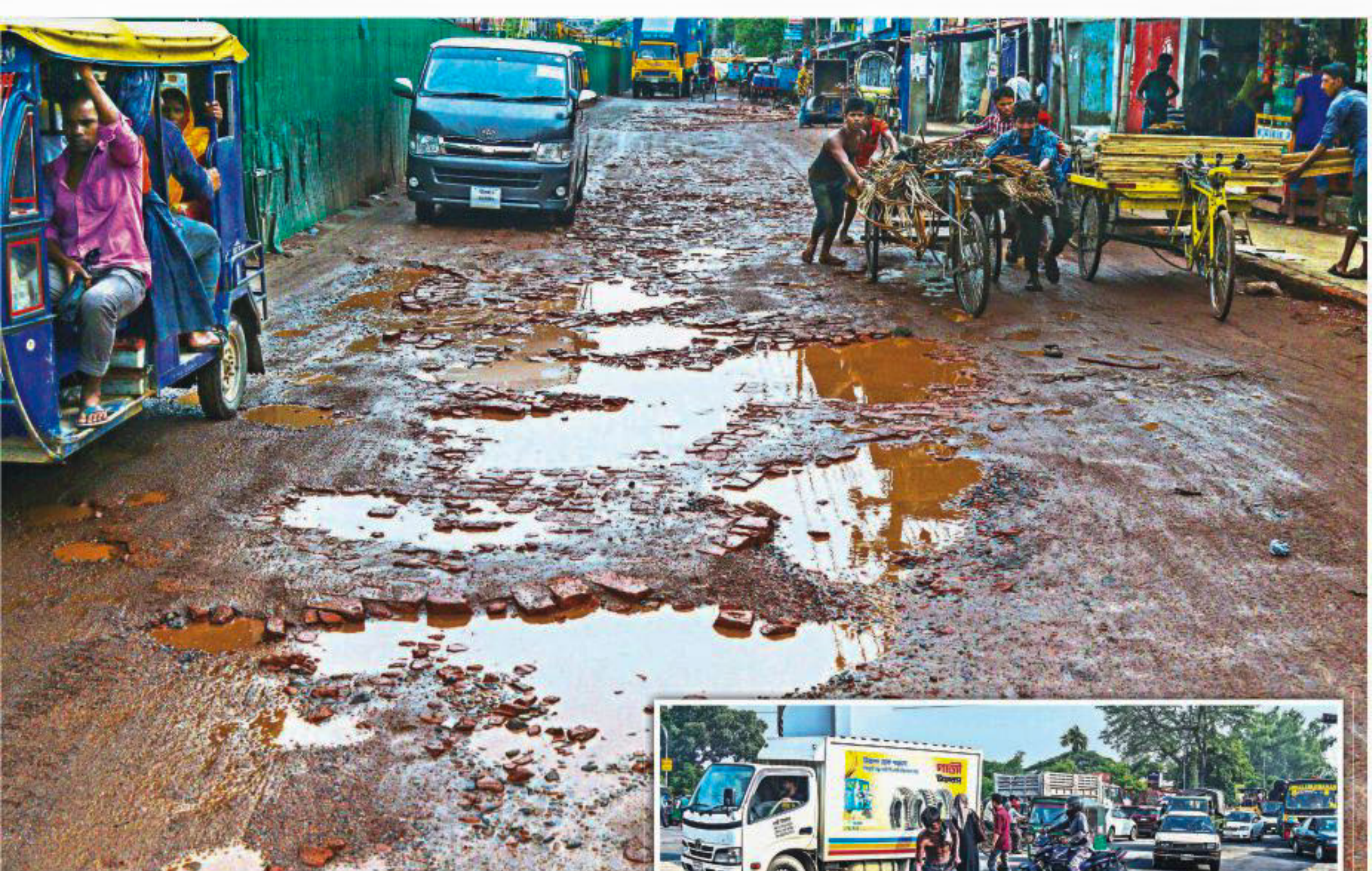
Many roads of Chattogram, like this one at North Patenga, have had their top layer scraped due to rain and waterlogging. City corporation authorities, however, have begun repair work at various points, such as Tiger Pass, inset.
