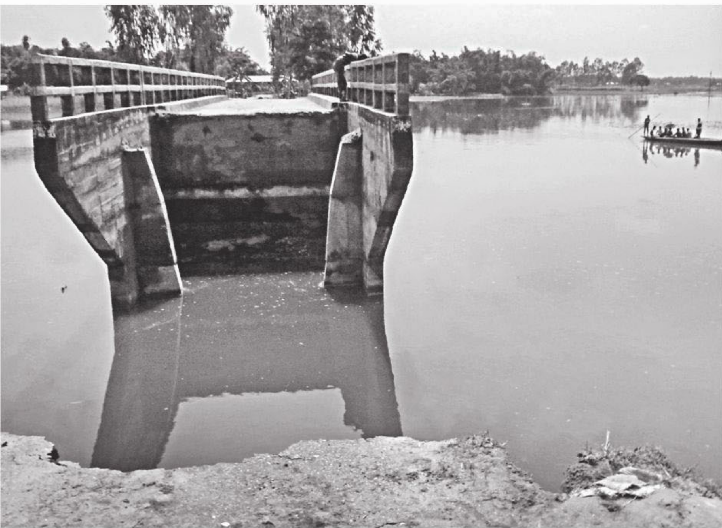
Left , the approach road to the bridge, which connects six villages in Jongra union with Patgram upazila headquarters of Lalmonirhat, was washed away by floodwaters on Sunday morning. Right , the damaged rail road between Gaibandha and Bonarpara section at Trimohoni in Gaibandha.
