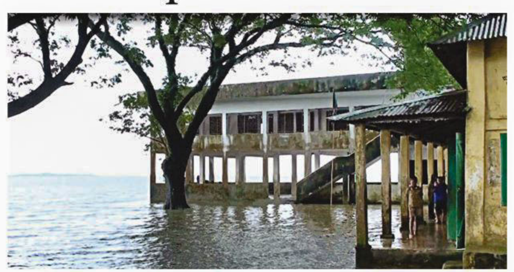
Inundated Sohona Government Primary School in Tahirpur.
