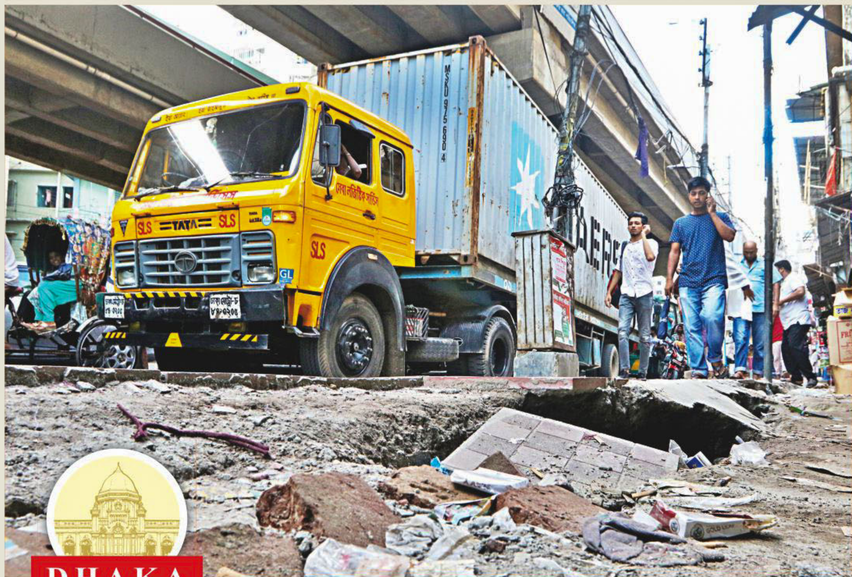
Tiles of the footpath are coming off, while the sloping cement covering of the drain underneath it is also crumbling. The photos were taken last week.
