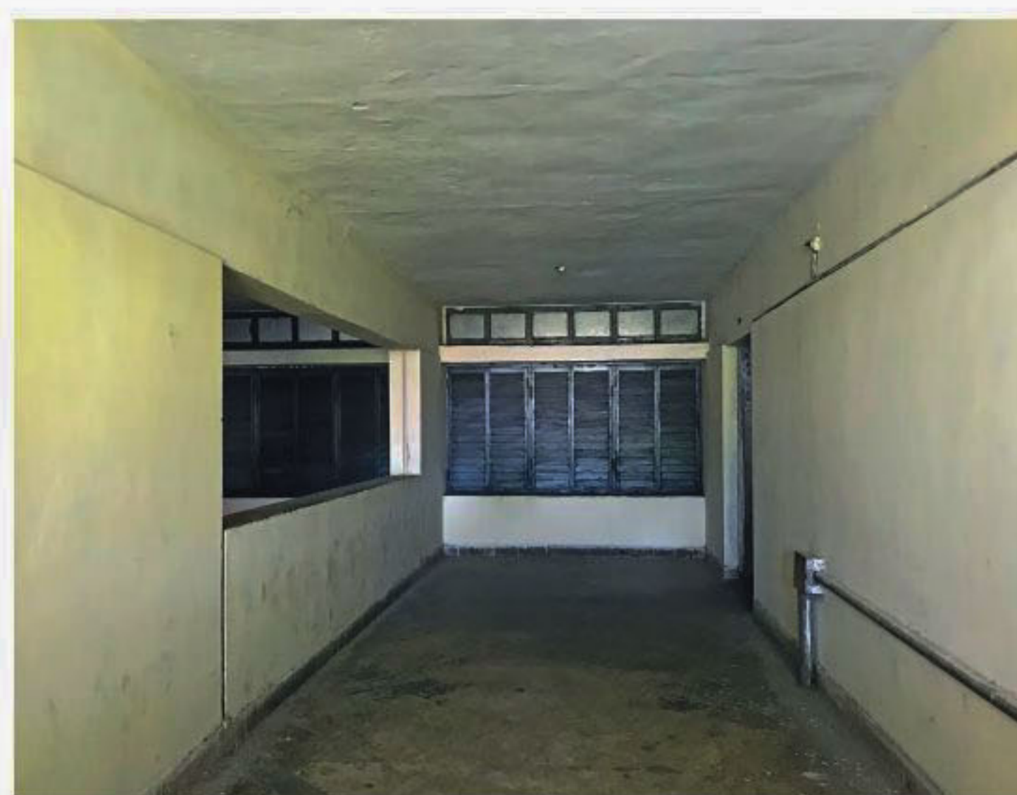
Additional space between classroom and corridor for meeting place, Sylhet Polytechnic Institute
