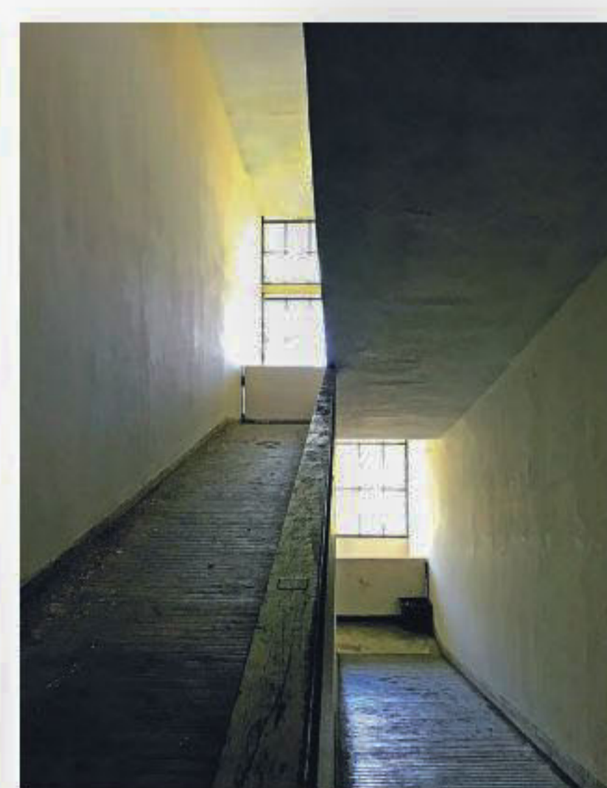
Use of ramp for vertical movement, Sylhet Polytechnic Institute
