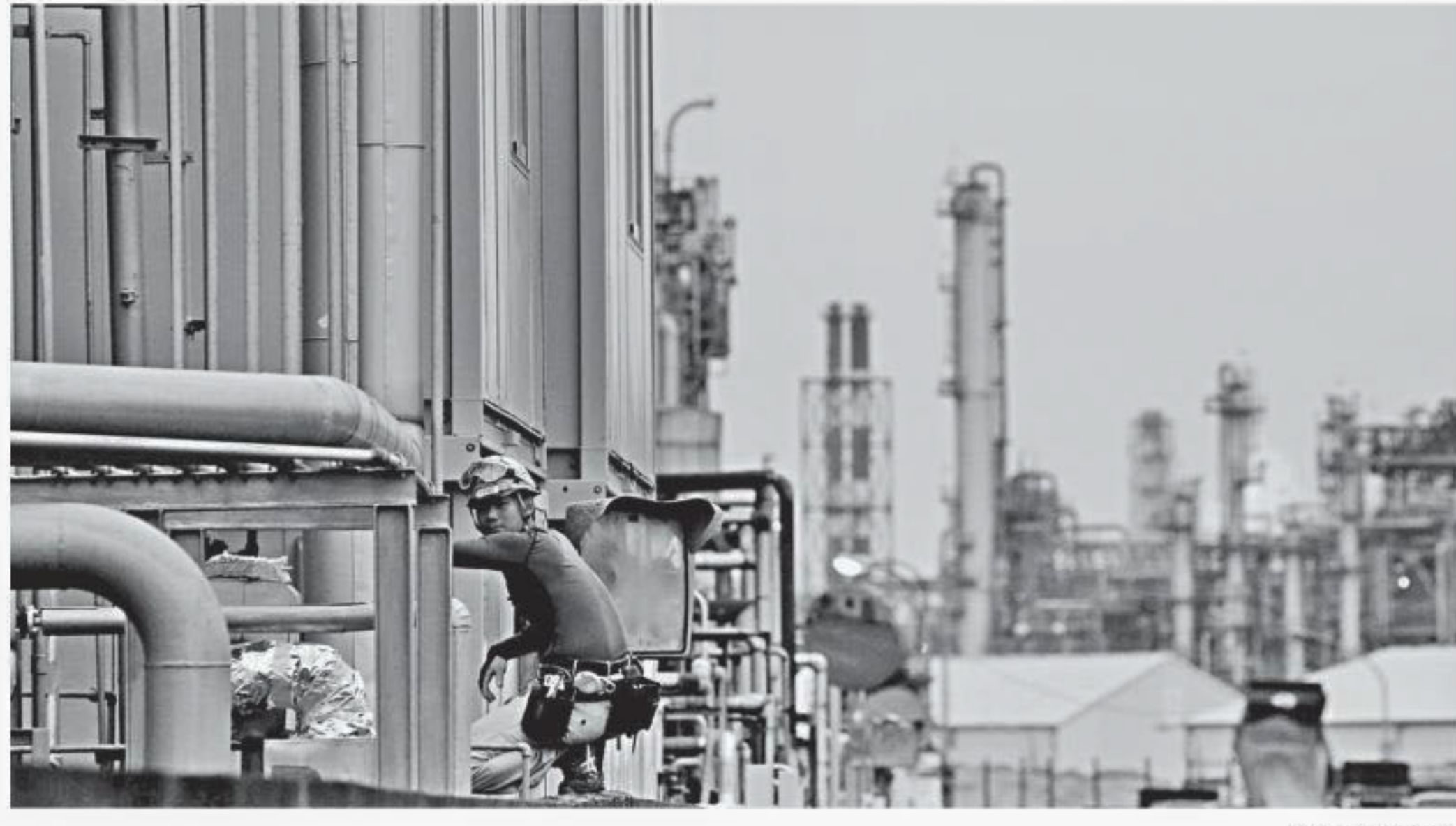
A worker is seen in front of facilities and chimneys of factories at the Keihin Industrial Zone in Kawasaki, Japan.
