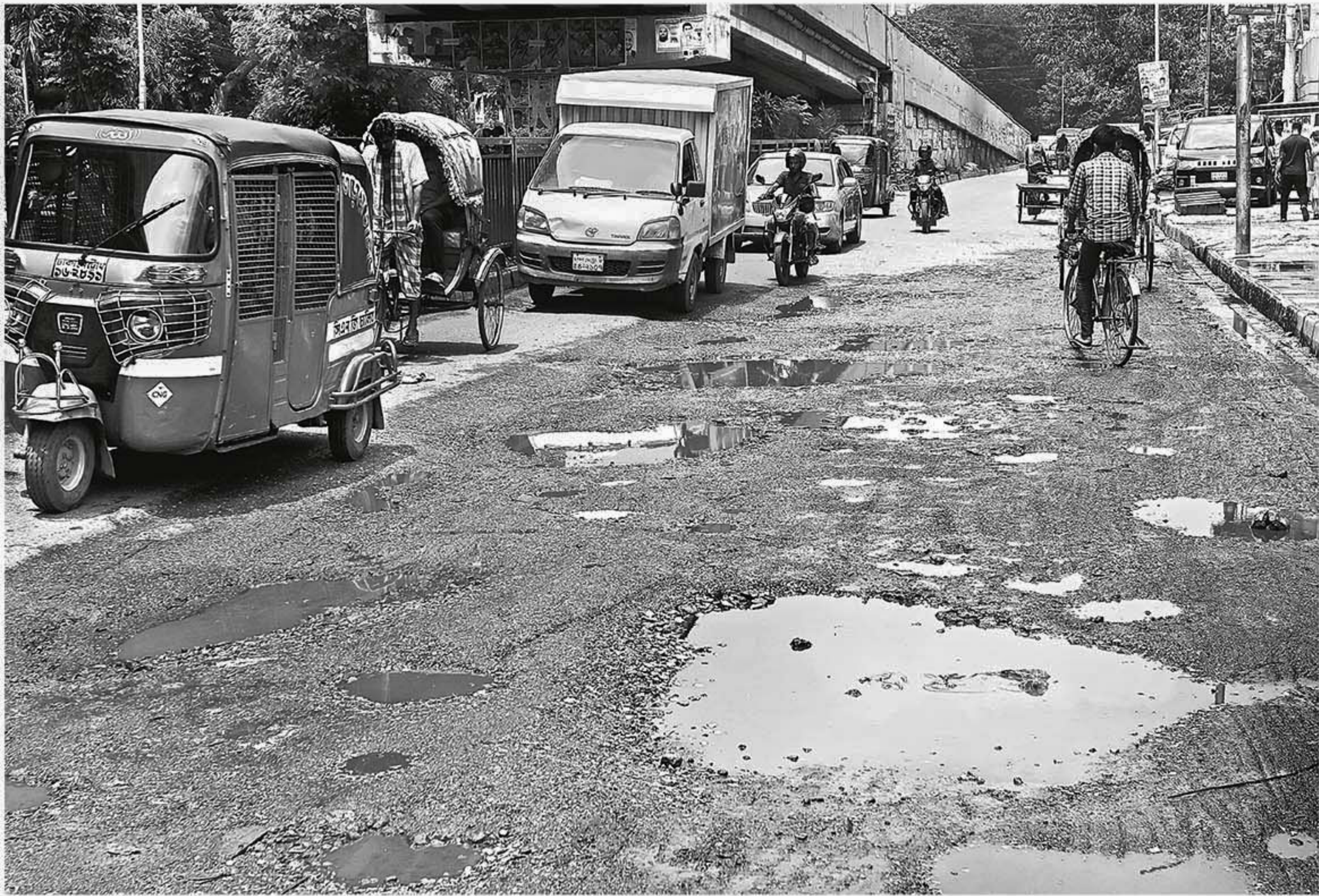
A part of Panthapath-Tejgaon link road in front of Karwan Bazar wholesale fish market is riddled with holes and puddles, limiting vehicle movement to just one lane. The photo was taken yesterday. PHOTO: PALASH KHAN
