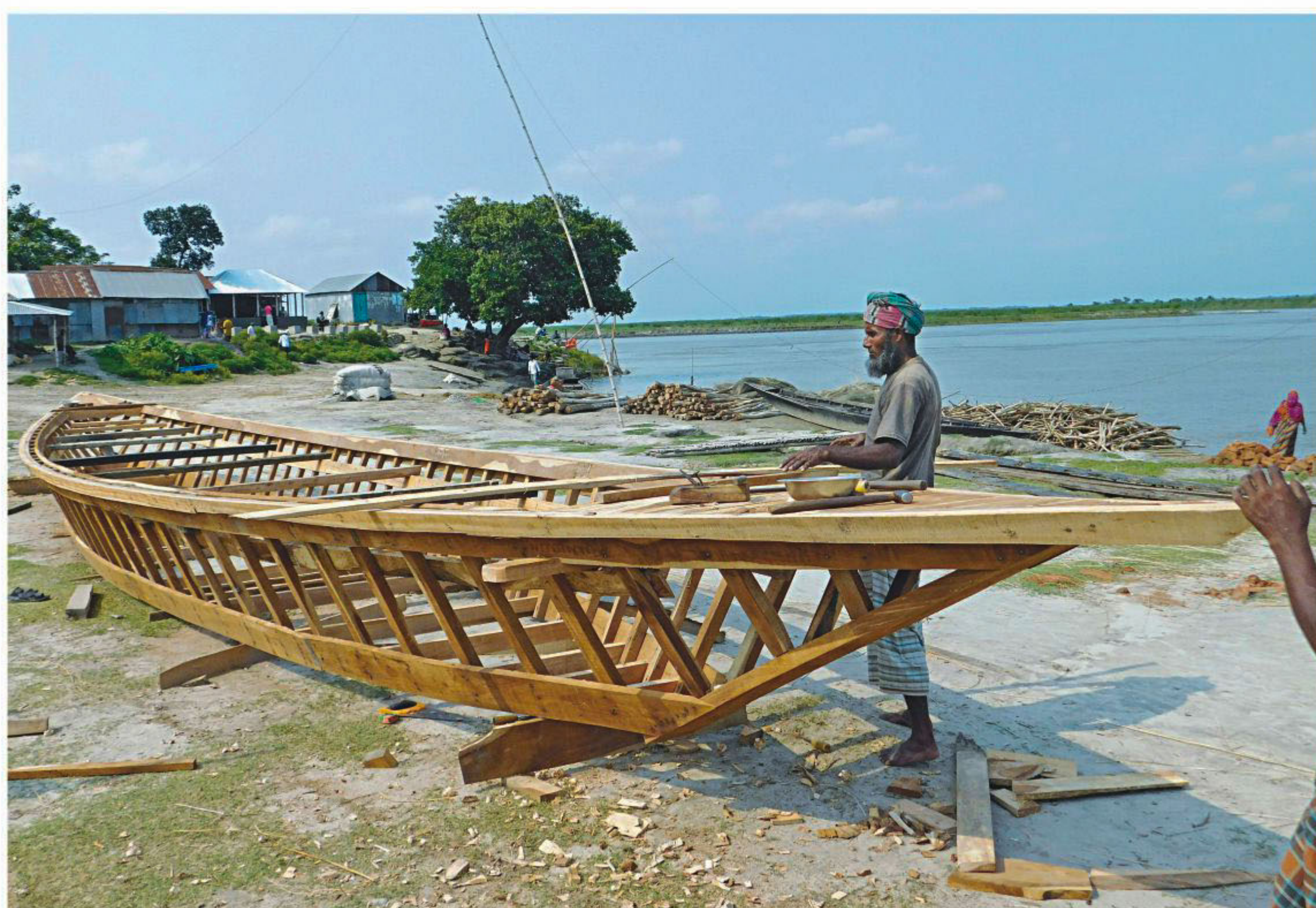
A new boat being built, an endeavour that can cost up to Tk 2 lakh, in preparation for the upcoming monsoon season. Almost 2,000 people -- especially those from the five nearby chars -- use such boats every day to cross the Jamuna river. The photo was taken from Bogura's Dhunat upazila recently.
