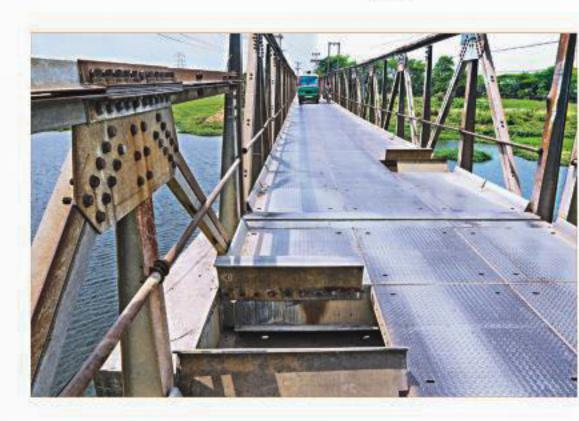
Truckers overloading their vehicles and getting on Bailey bridges is causing frequent collapse of the temporary structures, some of which are decades old.
