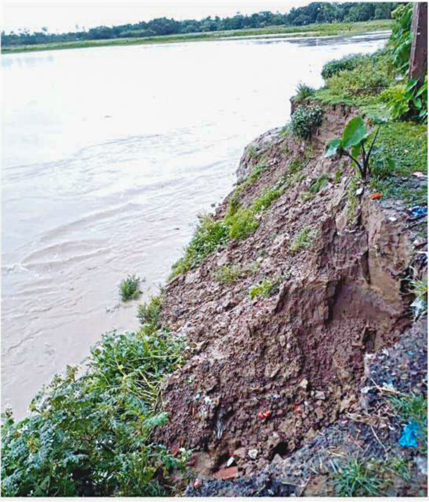
Rising level of water in the Monu river has been damaging different parts of its embankment in Moulvibazar. The photos were taken from in Moulvibazar 's Kulaura upazila yesterday.
