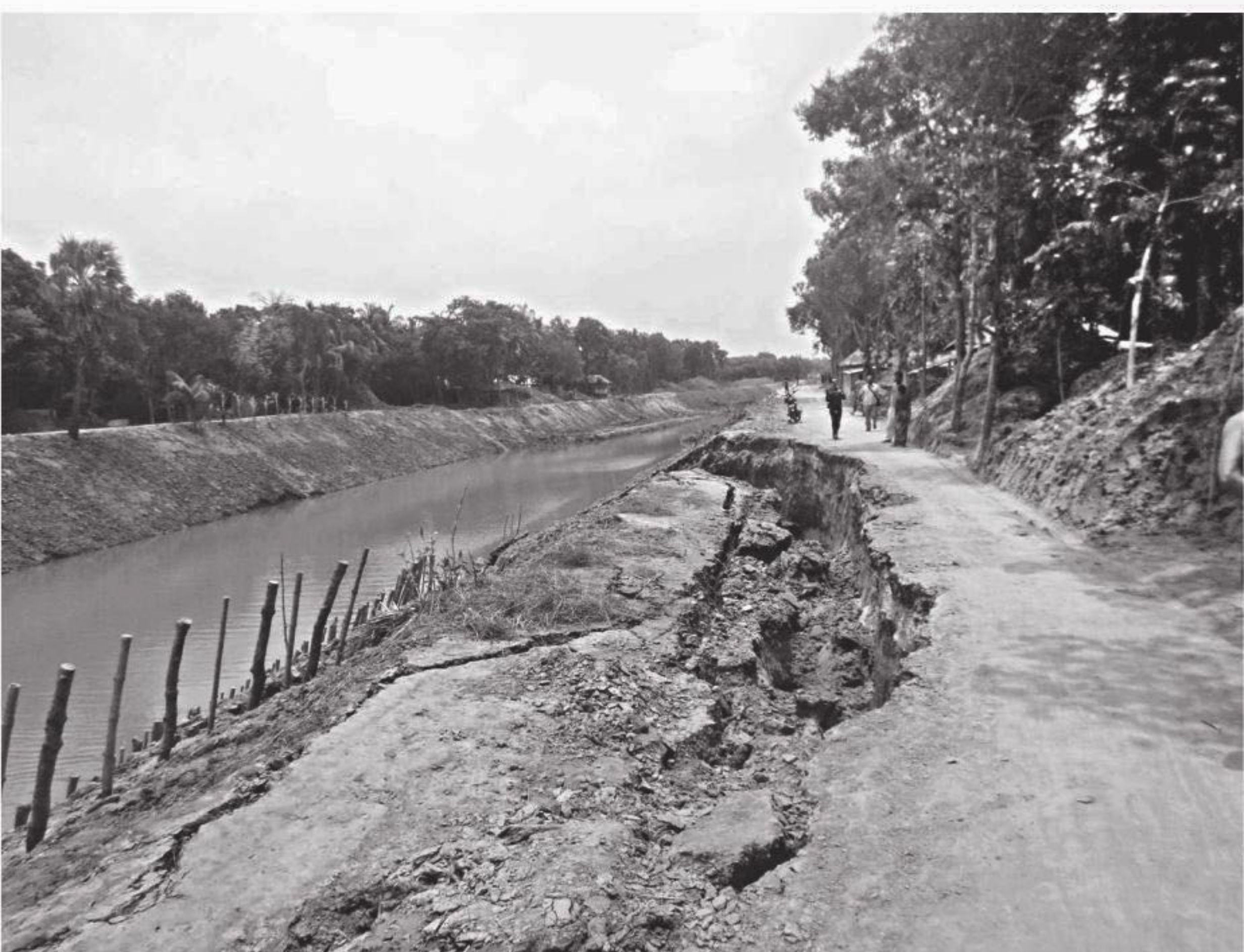
A 200-metre portion of Narua-Lalgolbad road has remained in an awful condition following collapse of the spot on the bank of the Katra river at Baksadangi village in Narua union of Rajbari's Baliakandi upazila a few days ago. Locals alleged that unplanned excavation of the river caused the problem.
