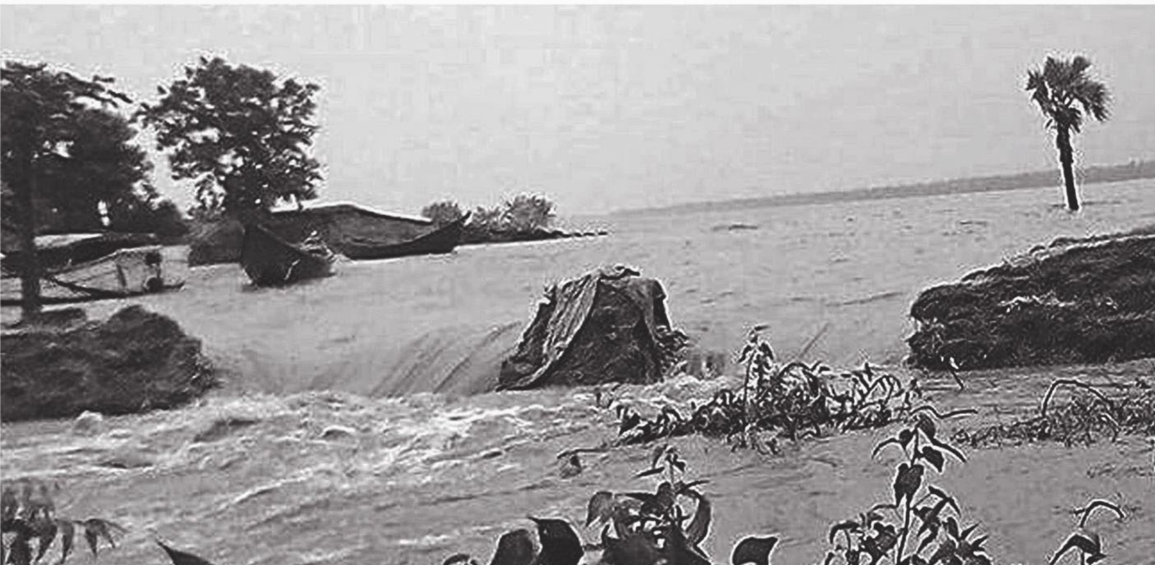
Water rushes in through the breached portion of the embankment on the Ramnabad river, flooding villages in Lalua union under Kalapara upazila of Patuakhali.
