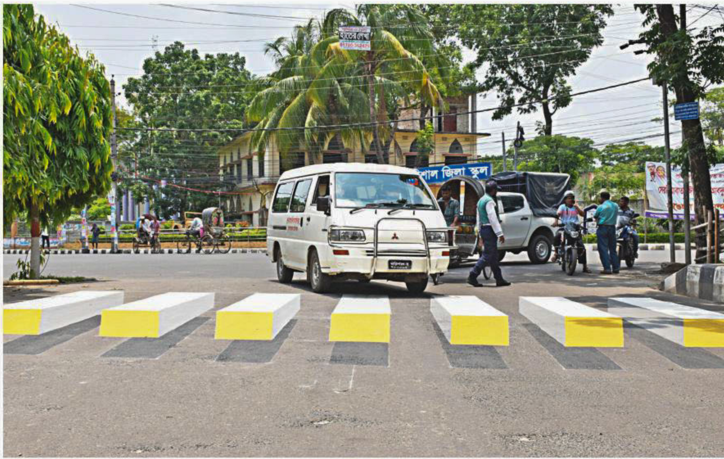
Although painted on a flat surface, this zebra crossing acts as a 3D optical illusion, prompting vehicles to slow down.
