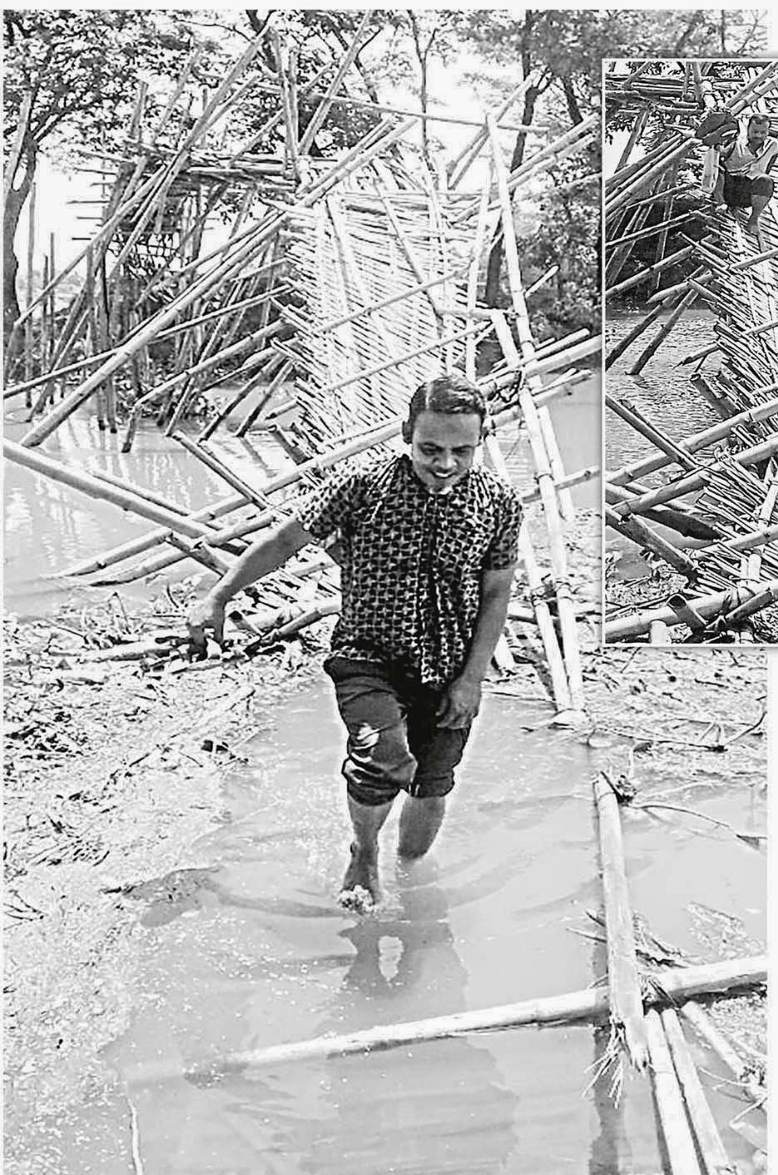
A man wades through ankle-deep water after crossing the collapsed bamboo bridge over the Bhogai river at Dakkhin Ranigaon village in Netrakona's Kalmakanda upazila. Inset, another man makes an arduous efforts, defying the risk of accident, in case he slips from the steep deck of the twisted structure as the alternative way of crossing the river seems a bit time consuming to him.
