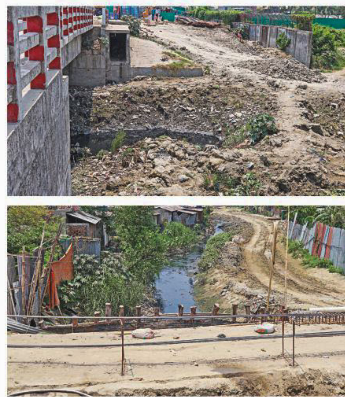
Under a project to ease waterlogging, temporary dams have been built on the canals that connect to Karnaphuli river. But these dams will stop rainwater from reaching the river quickly, making waterlogging much worse. The bottom right photo shows the connecting point between Tekpara canal and the river, while the rest are of Kalabagicha. The photos were taken yesterday.
