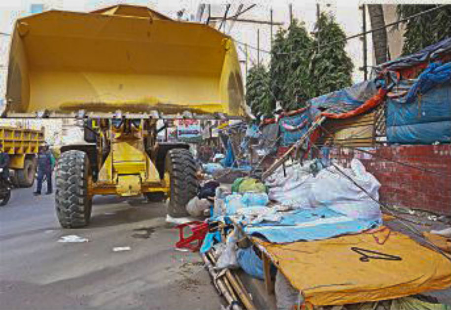
Bulldozers razing the Gulistan sidewalks in 2017
