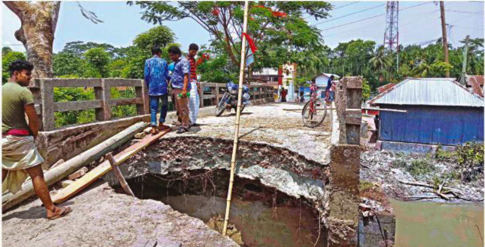
The approach road of the bridge on Indurkani-Bagolerhat road adjacent to Pattasi Bazar in Indurkani upazila of Pirojpur started subsiding on Monday and finally got separated from the bridge yesterday, hampering road communication with the upazila headquarters.
