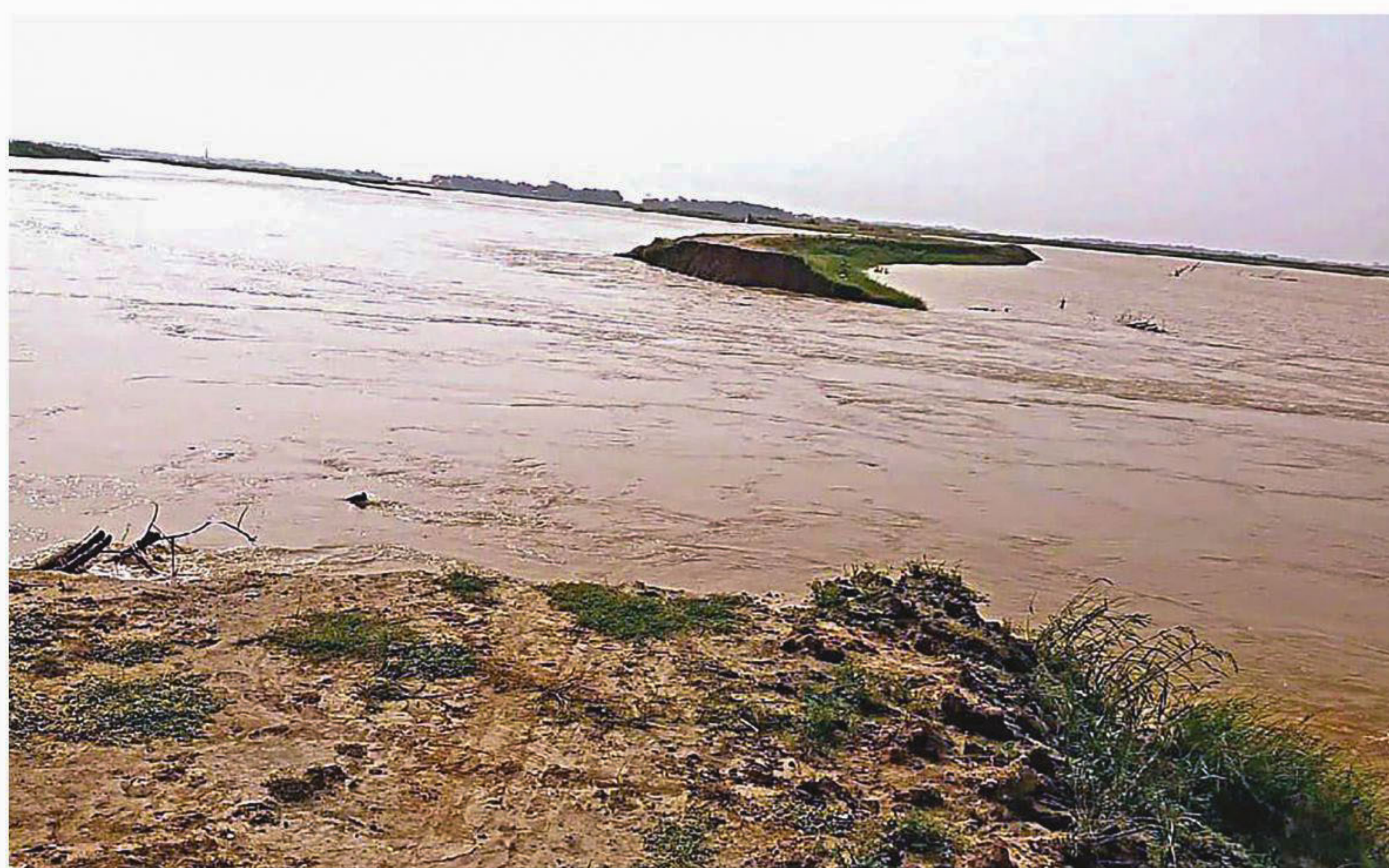
This embankment on the Guraduba haor in Dharmapasha upazila of Sunamganj collapsed early yesterday, inundating nearly ripe Boro paddy on hundreds of acres of land in adjacent Borokhapon union under Kalmakanda upazila of Netrakona.
