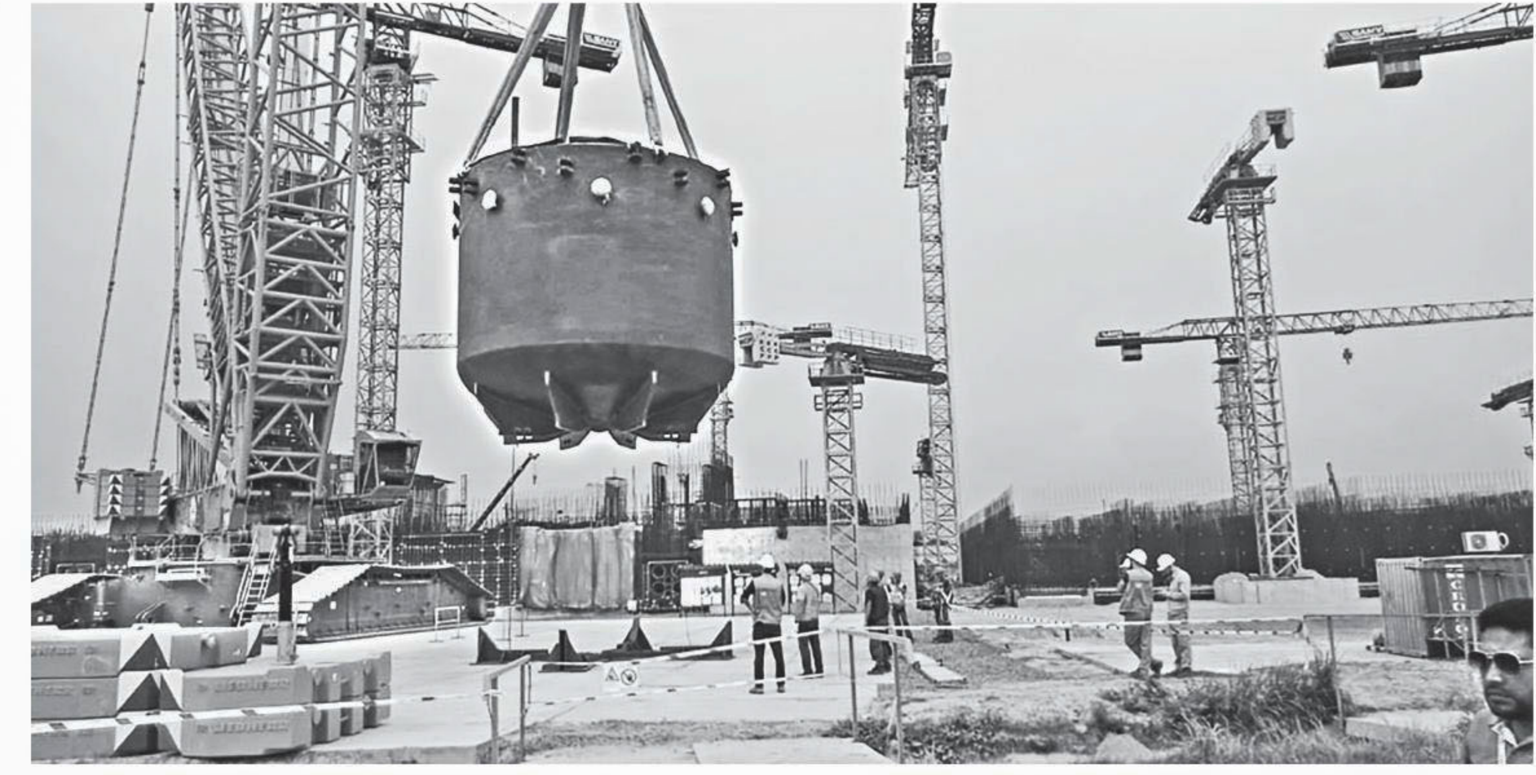
Installation of “core catcher”, a device for catching molten core (active part of the reactor that contains nuclear fuel), began at unit 2 of Rooppur Nuclear Power Plant yesterday. Science and Technology Minister Yeafesh Osman inaugurated the work in the morning.
