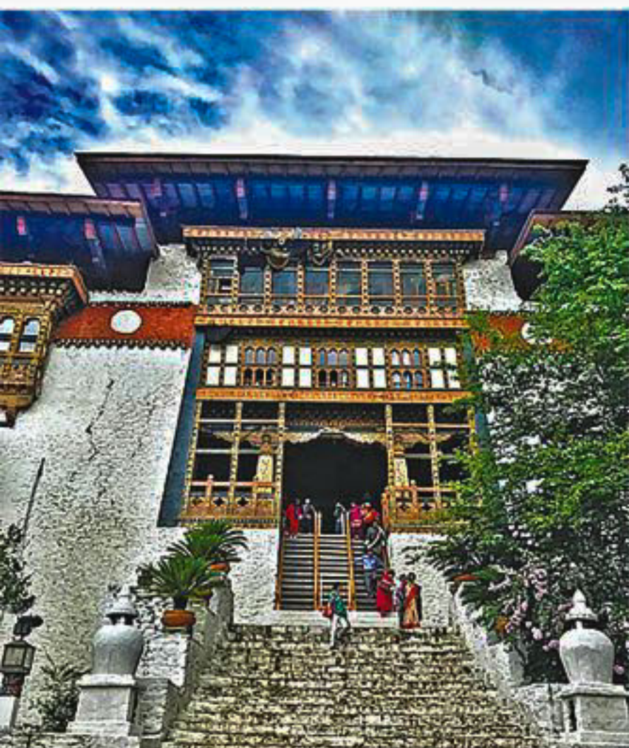
The entire structure of the Punakha Dzong is breathtakingly beautiful.
