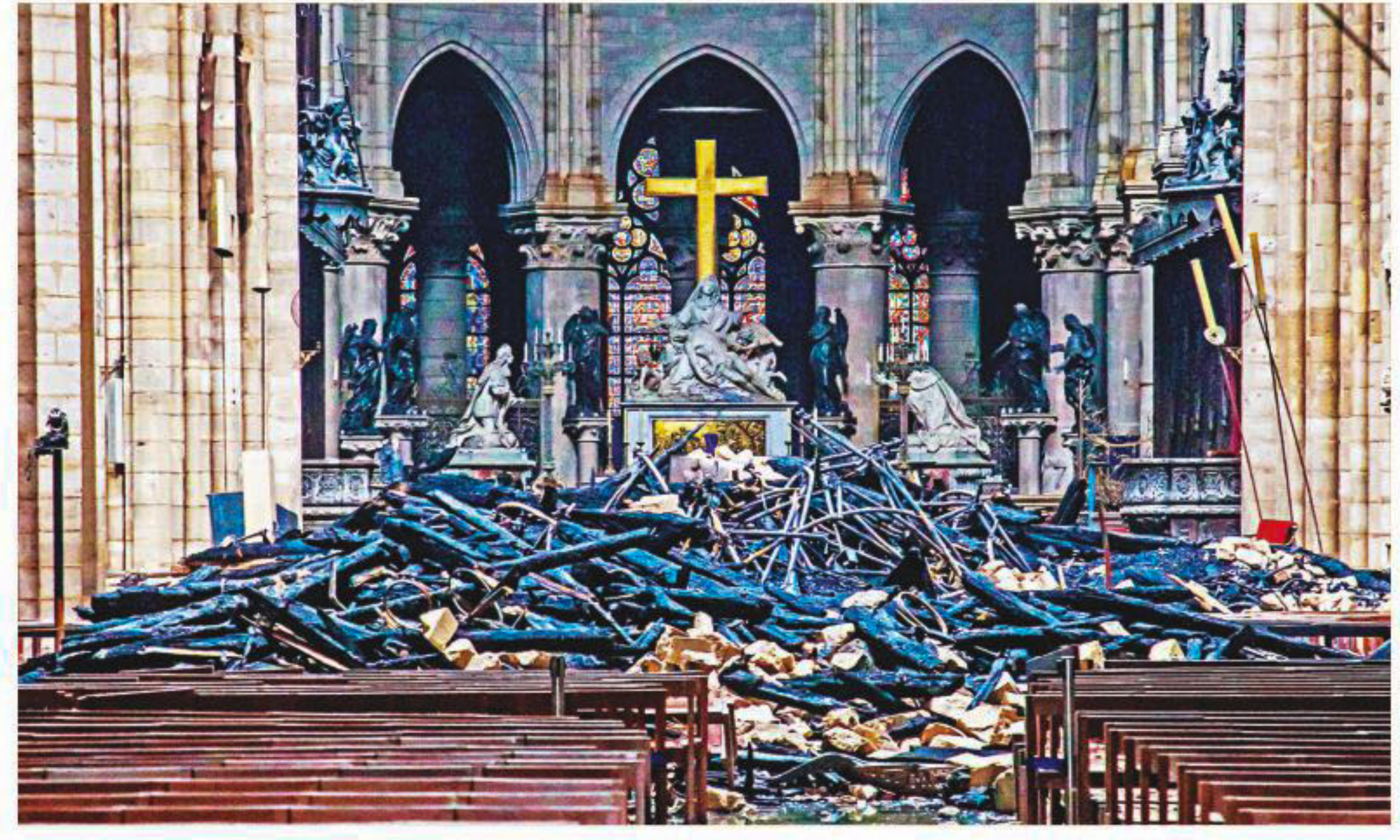
This general view shows debris inside the Notre-Dame Cathedral, on Tuesday.
