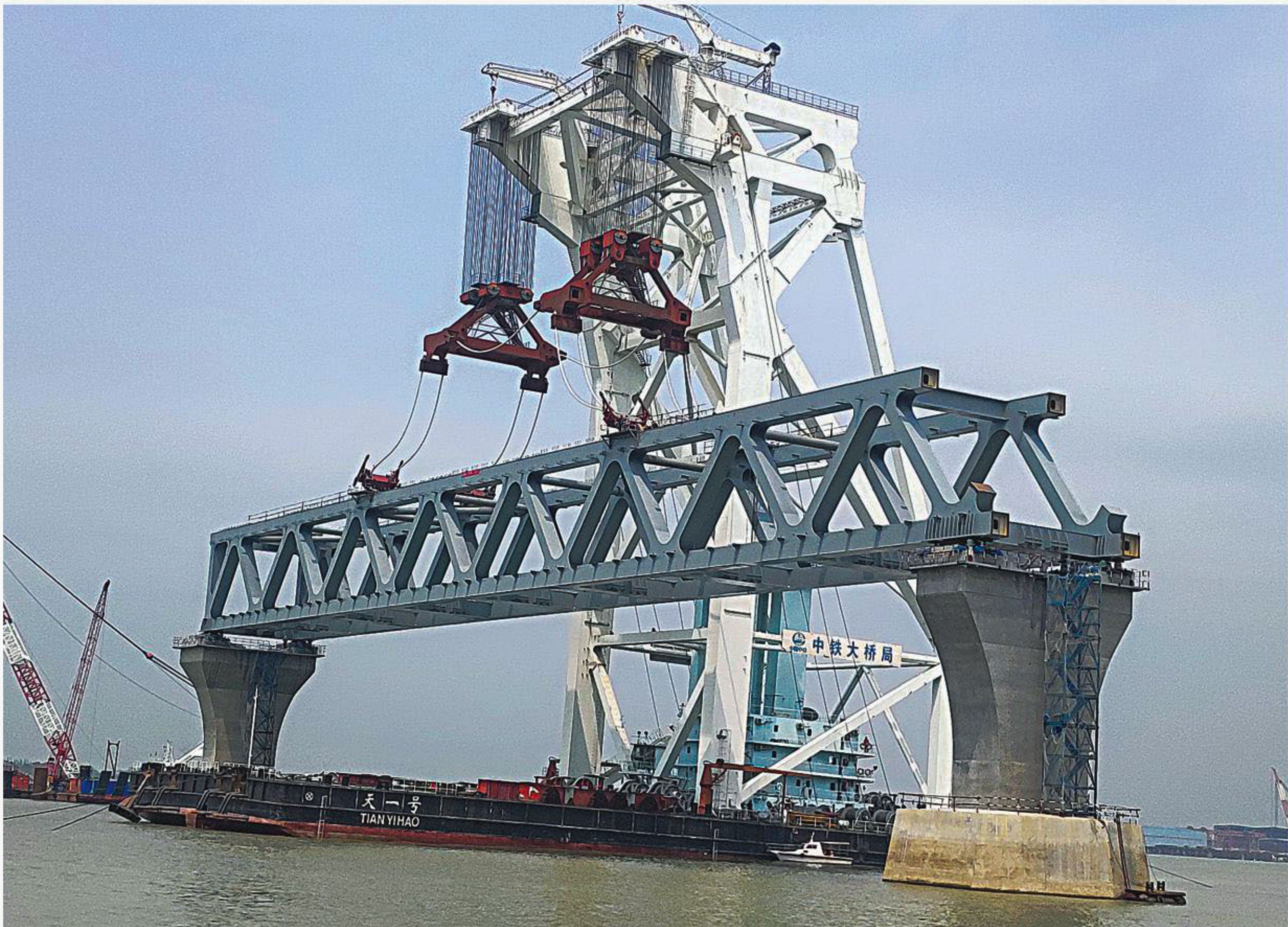
A crane placing a span of the Padma bridge on two pillars off Munshiganj's Mawa. The picture was taken yesterday.
