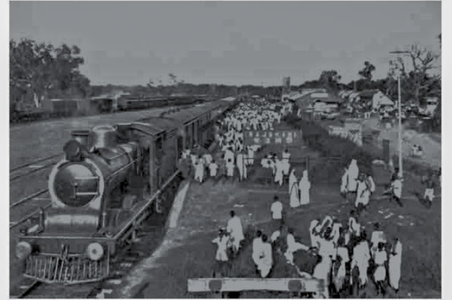
PHOTO: CHRIS WALKER COLLECTION/THE RESTORATION & ARCHIVING TRUST A train waits at the Rajshahi station in the 1930s.
