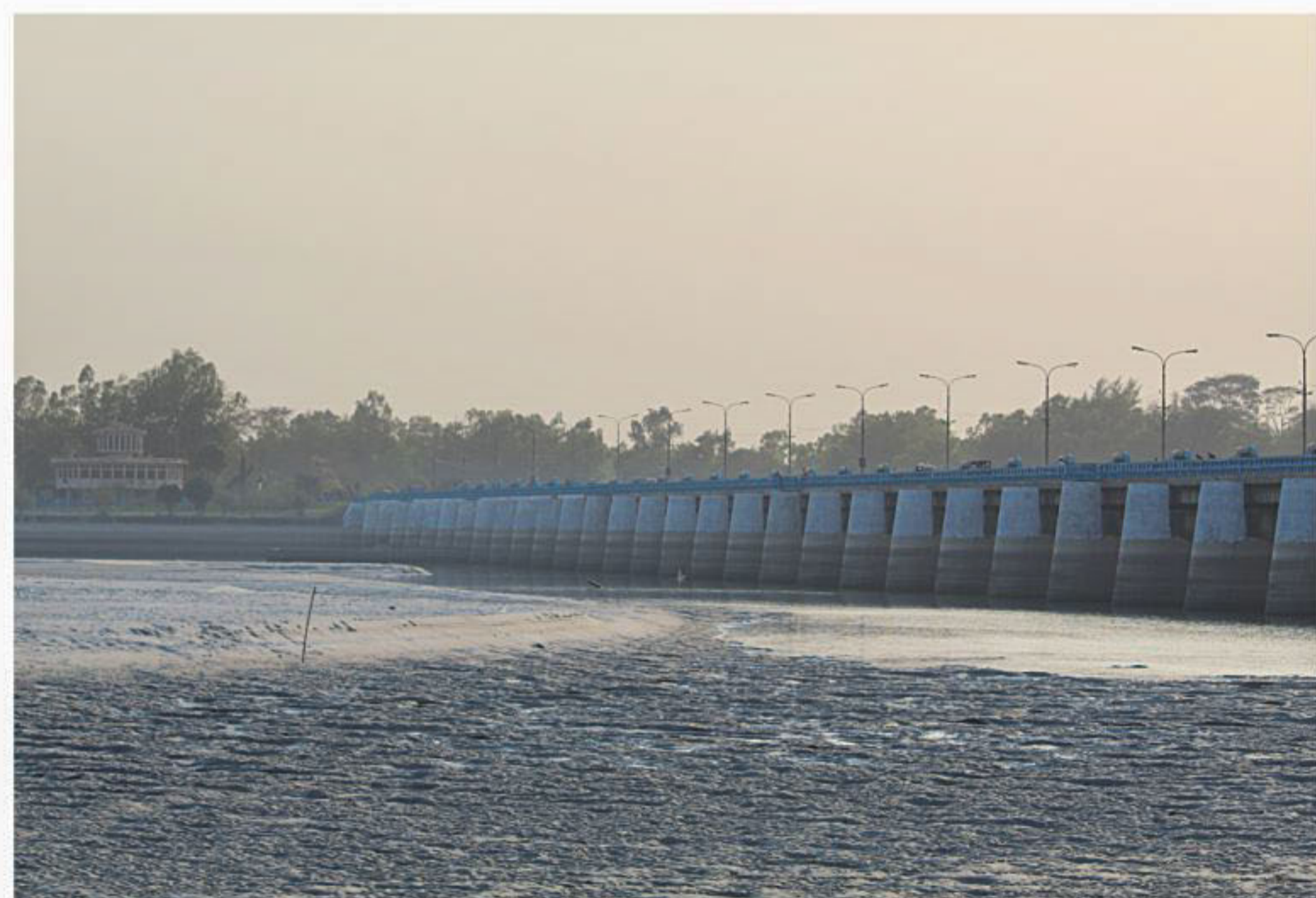
Accumulation of sediment on the downstream of Teesta river is choking the freshwater ecosystem.
