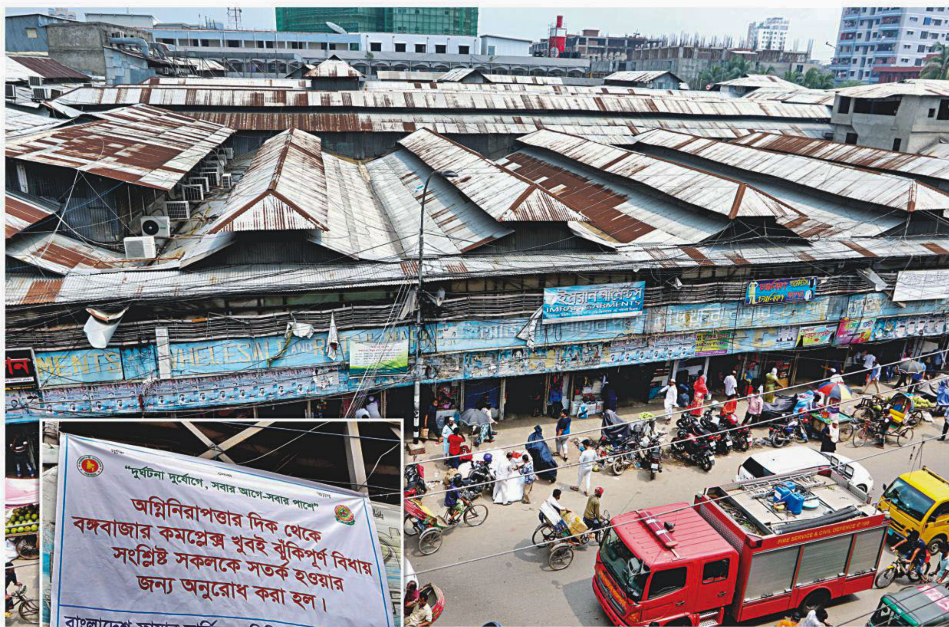
The congested multi-storey apparel market Bangabazar in the capital is one of the shopping centres marked risky, inset, by the fire department. The pictures were taken yesterday morning.
