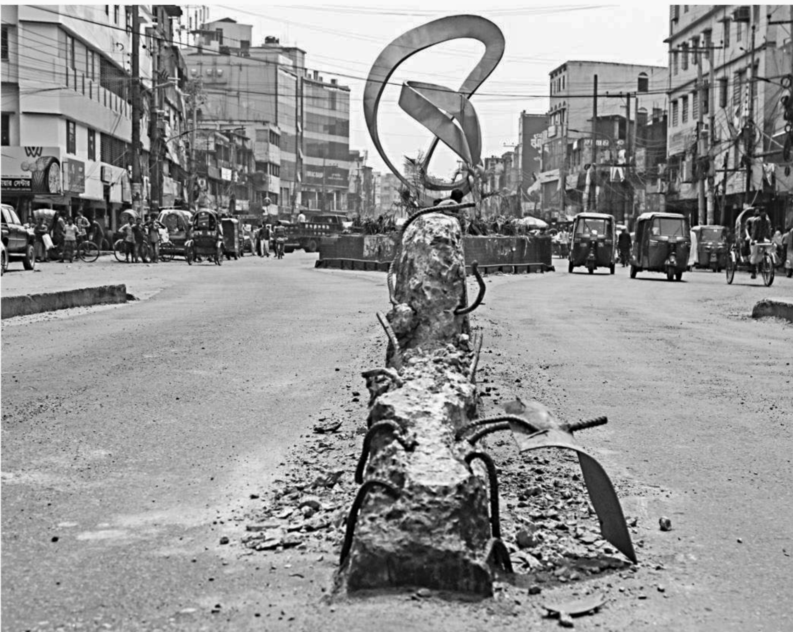
This damaged road divider, with rods sticking out, could cause an accident to approaching vehicles. The photo was taken on Dewanhat overpass in Dhaniala area of Chattogram city yesterday.
