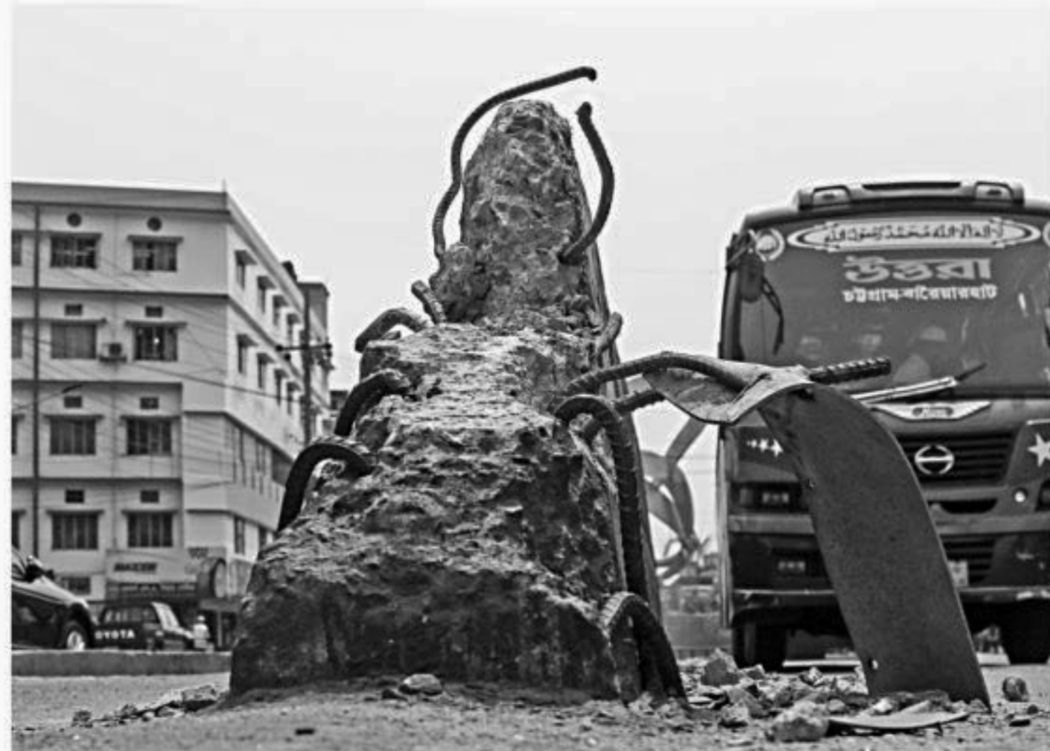
This damaged road divider, with rods sticking out, could cause an accident to approaching vehicles. The photo was taken on Dewanhat overpass in Dhaniala area of Chattogram city yesterday.
