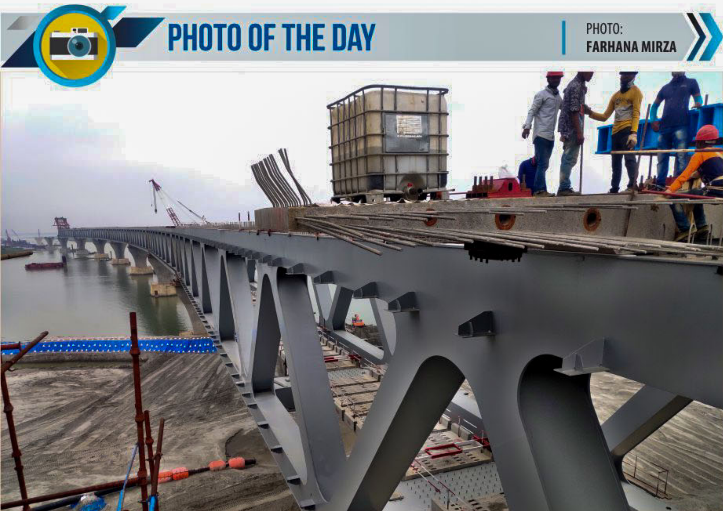
The first roadway slab being installed on the Jazira end of the Padma bridge in Shariatpur. The 2 metres in width and 22 metres in length slab was placed on the "7-F" span between pillar 41 and 42 yesterday. A total of 2,931 slabs will be set up on the 6.15km bridge.
