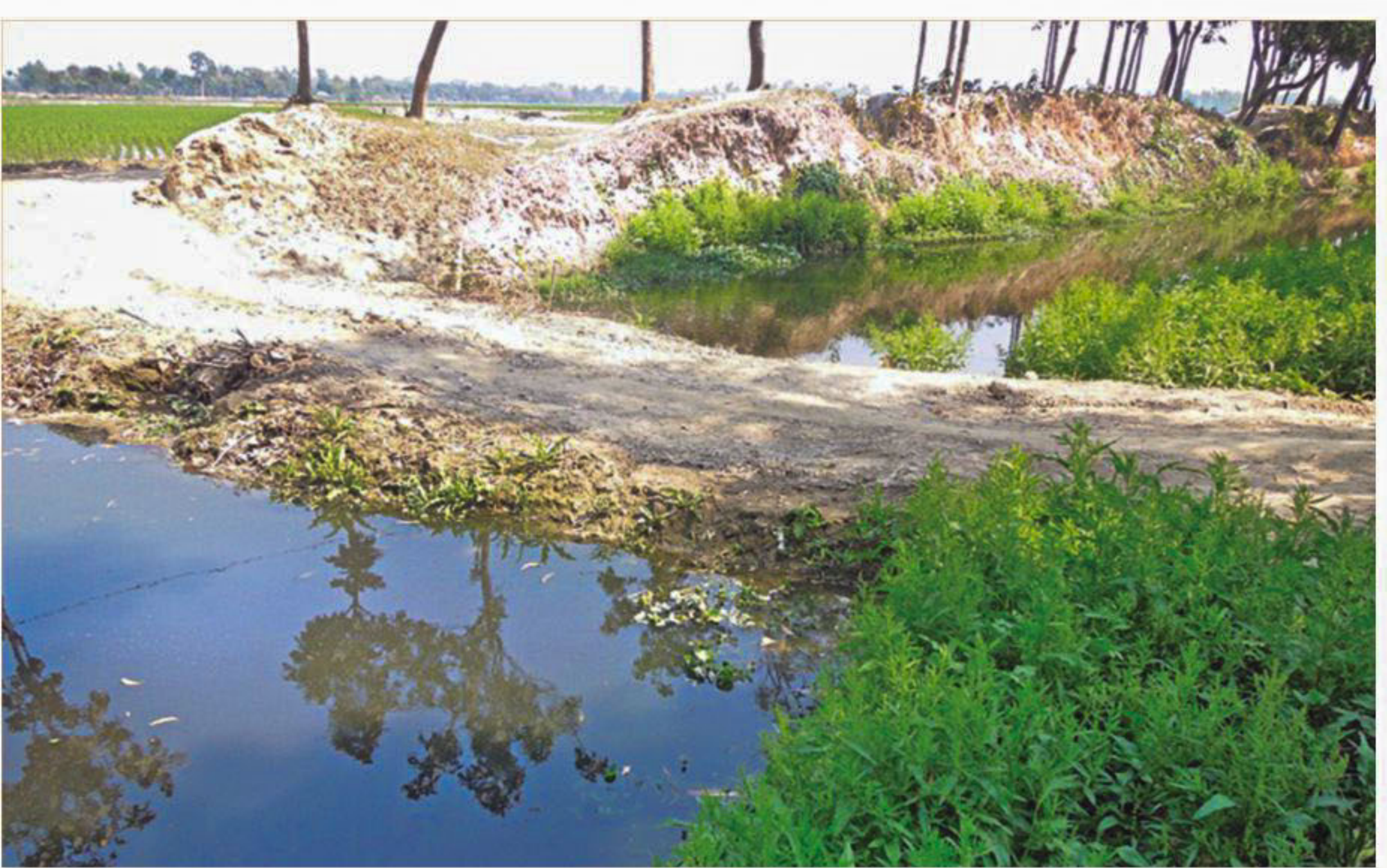
This earthen road has been built across the Water Development Board's canal at Pathan Para village in Nilphamari's Saidpur upazila, obstructing the flow. PHOTO: EAM ASADUZZAMAN
