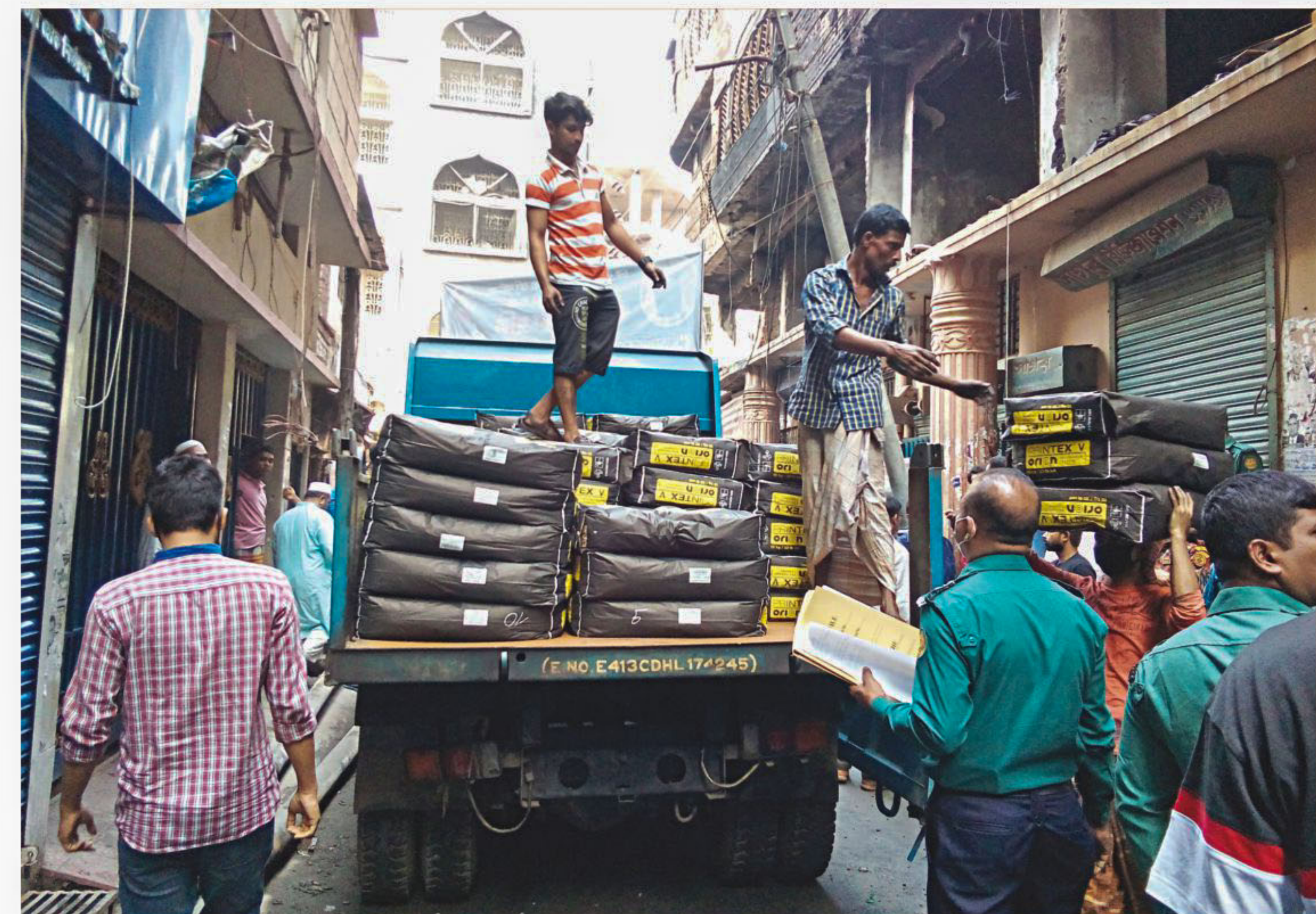
Bags of chemical substances stockpiled in the basement of Haji Wahed Mansion in the capital's Chawkbazar are being removed from the building by Dhaka South City Corporation yesterday.
