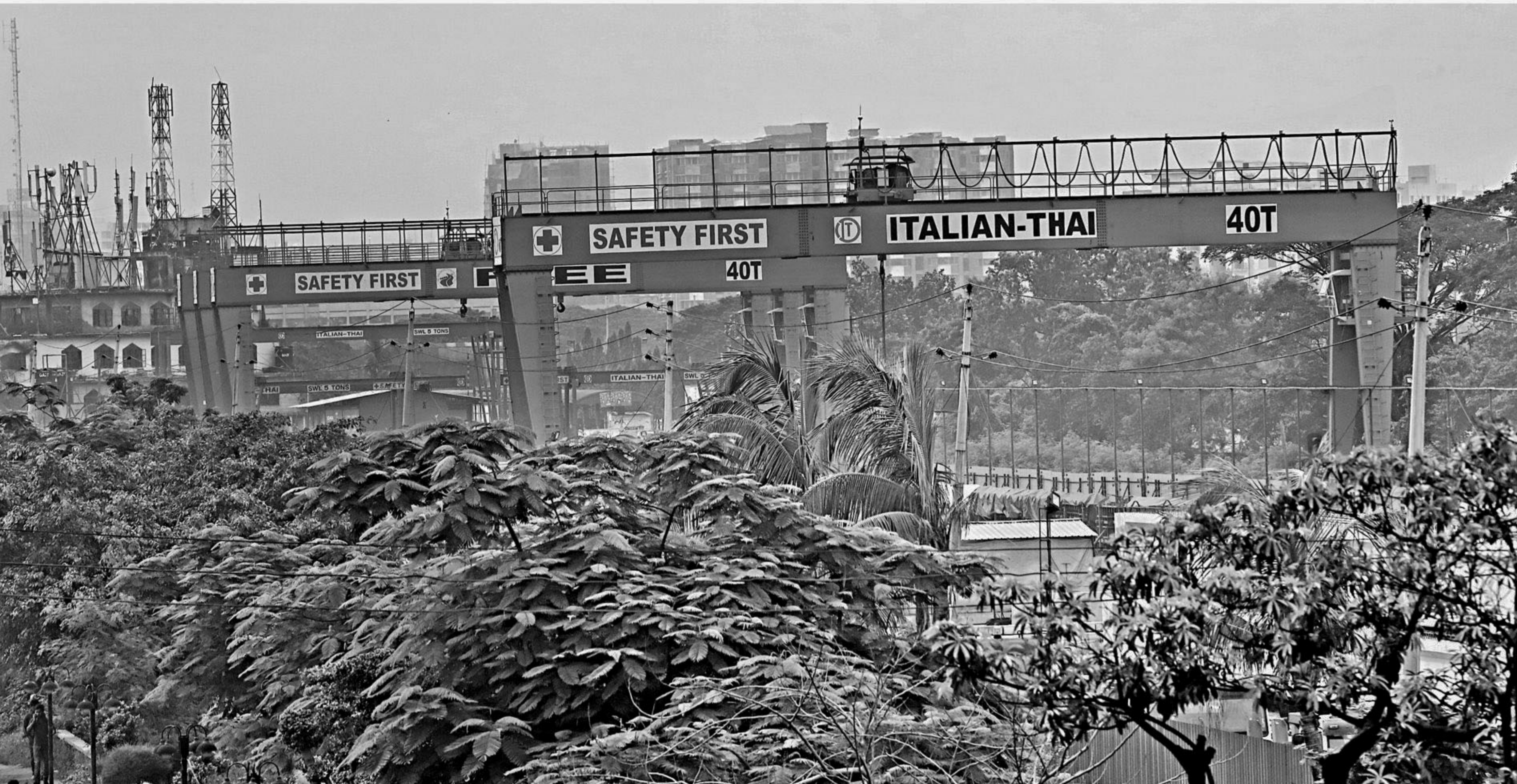
Elevated Expressway construction at Airport Road.
