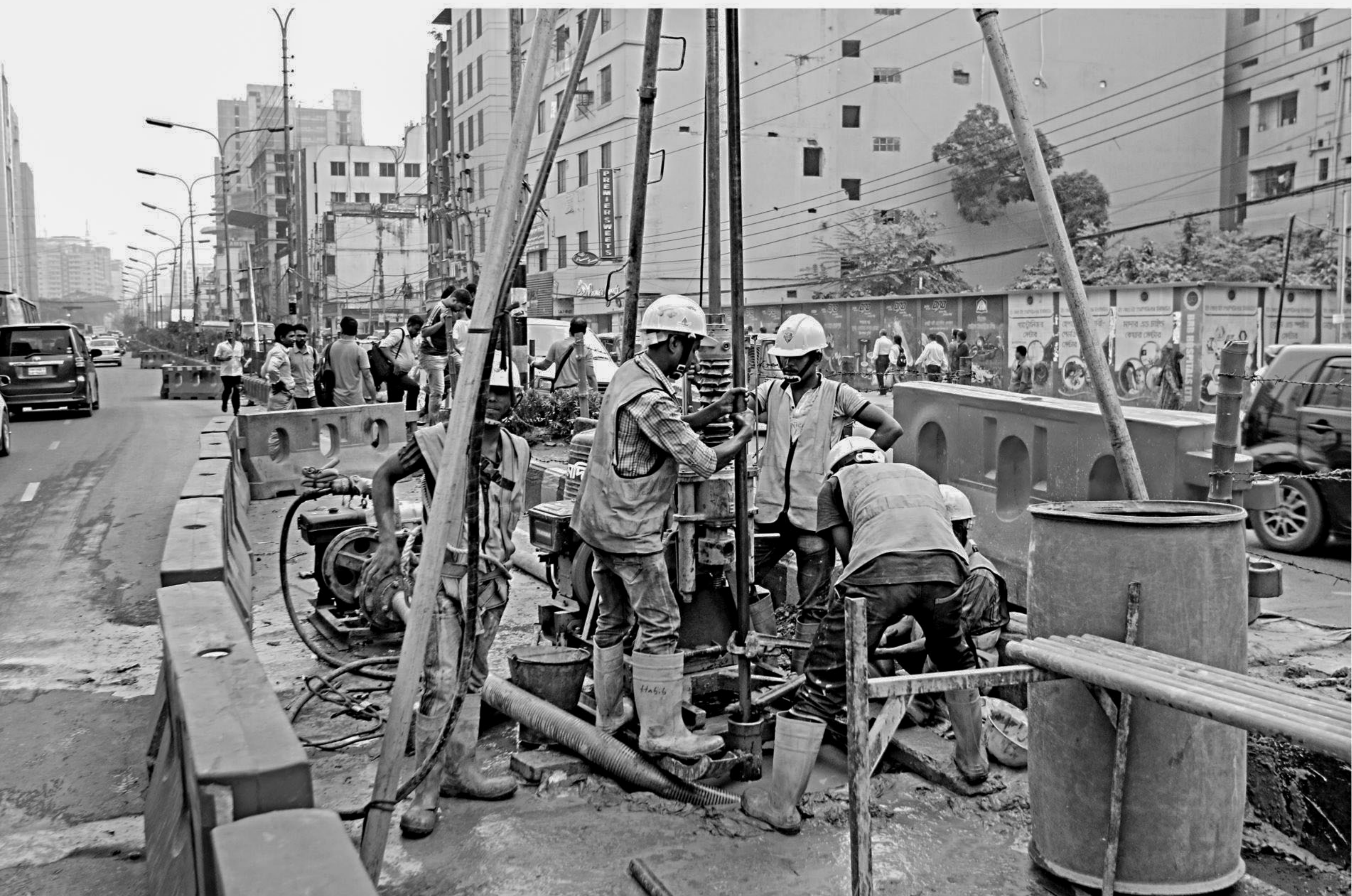
Metro rail construction in Kazi Nazrul Islam Avenue.
