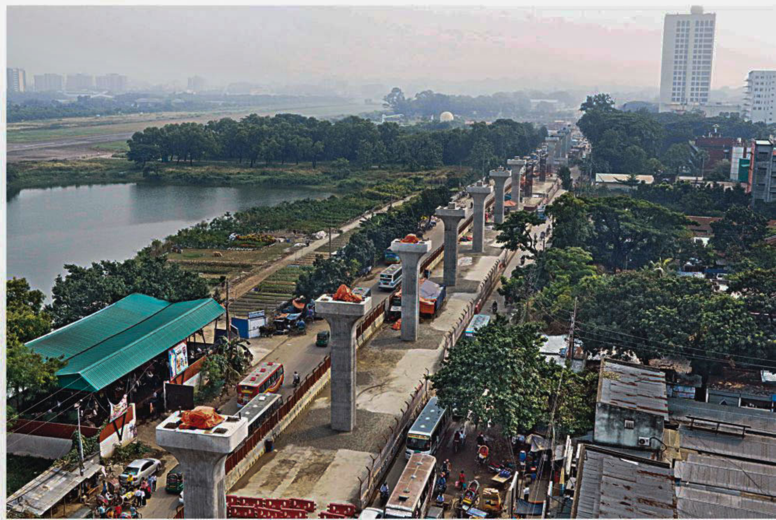
Metro rail construction, Rokeya Sharani.
