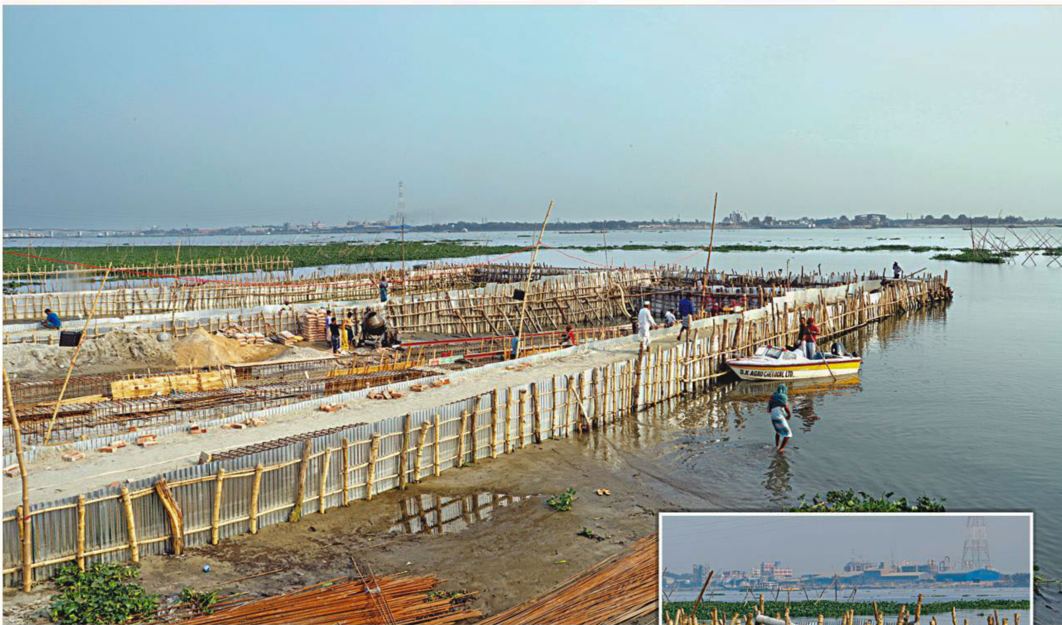
A private firm has put up a makeshift enclosure to build two slipways after encroaching into the Meghna river in Gazaria of Munshiganj. Inset, water being pumped out from the enclosed area. The photos were taken a few days ago.
