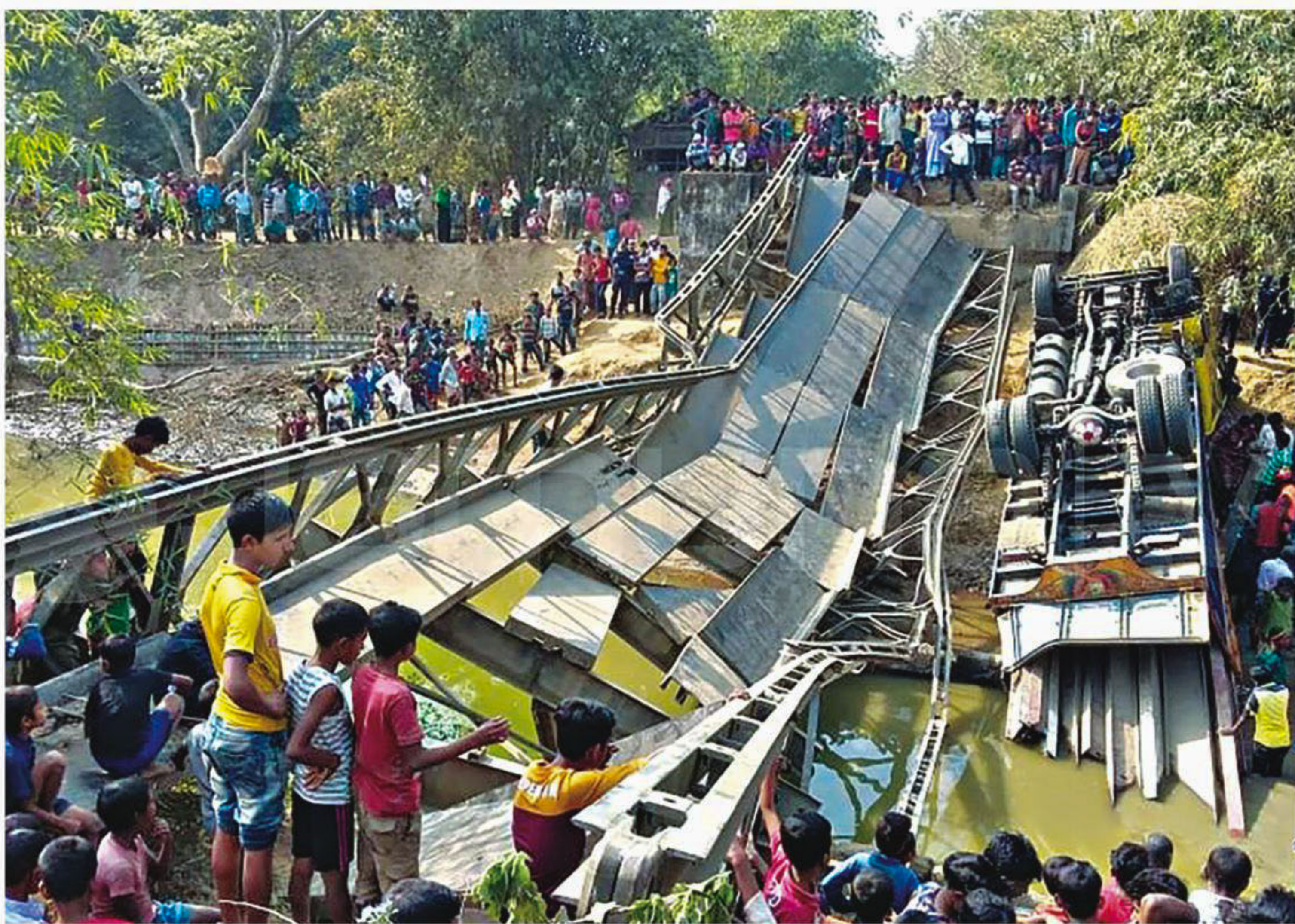
This Bailey bridge collapsed when an overloaded truck was crossing it in Sunamganj's Bishwambarpur upazila yesterday. Two people in the truck were killed.
